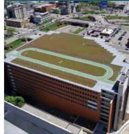
process, which uses concrete mixtures with low water-to-cementitious ratios (0.32 – 0.40) and is easier to provide for appropriate curing procedures. This results in higher-quality concrete with compressive strengths of at least 5000 psi, lower permeability, and hence greater overall durability. This will contribute to increasing the service life of a parking structure, while reducing maintenance costs.
