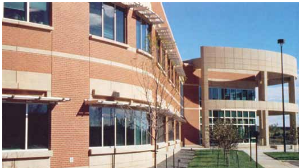
At the Jefferson County District Attorney's Office Building at Golden, Colo., the use of curved precast panels allowed the designers to repeat the radiused building corner with a curved open pergola at the entry. (Courtesy Jun Xia, Gensler)
