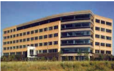
The use of curved precast panels allowed the designers to "break out of the box" at the 370 Interlocken Boulevard project in Broomfield, Colorado. (Courtesy Ed Lacasse)
