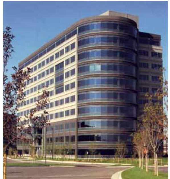
The combination of radiused structural precast panels and storefront glazing allowed designers to express a curved “glass” volume without the additional cost of the curtain wall at the 380 Interlocken Crescent project in Broomfield,
