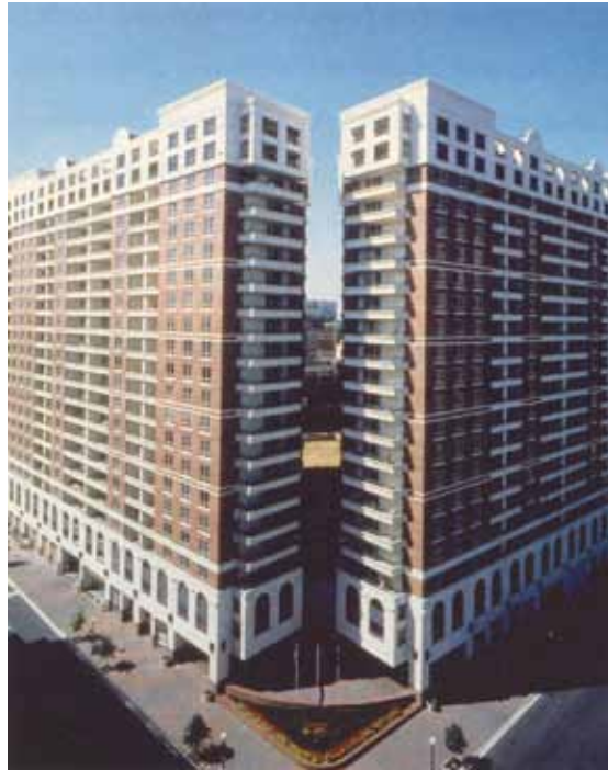
Lincoln Towers in Arlington, Va., was designed with precast window wall panels at the base of the building, incorporating arches, reveals and projections to articulate the elements. Precast concrete also is featured significantly at other openings in the façades, such as the balconies and windows at the top of the building. The precast used with masonry in this project adds interest and color to the project.
