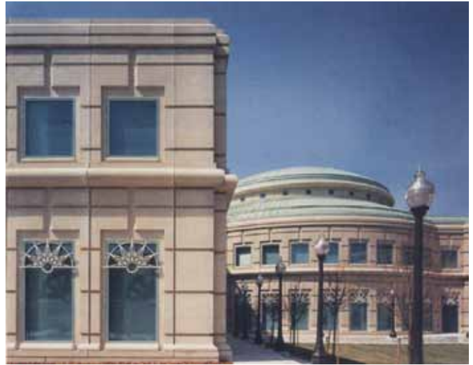
The courtyard space of the Aurora Municipal Justice Center indicates the interplay of both vertical and horizontal reveals with the building forms.
