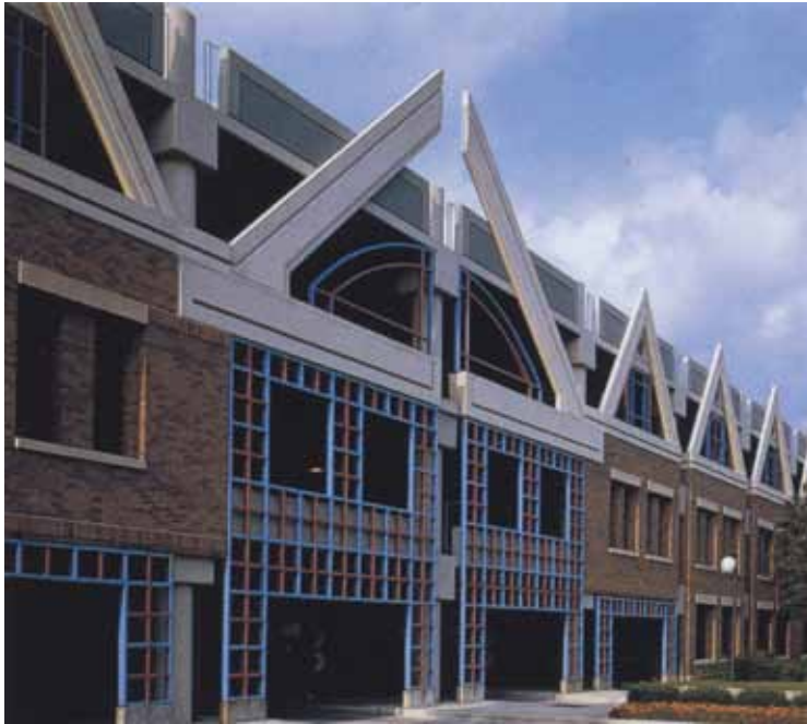
Holley Court Parking Facility in Oak Park, Ill., features precast concrete details that add both character and interest to the cornice and façade. The goal was to suggest residential rowhouses rather than a parking structure. (Courtesy ©Steinkamp/Ballog Chicago)
