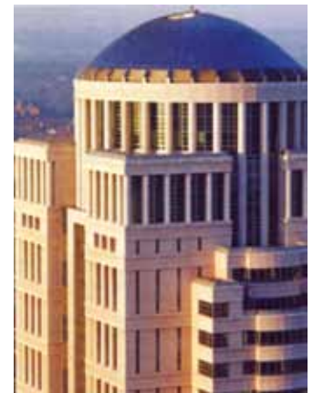
Recessed windows with columns, deep sills and soffits are used throughout.
