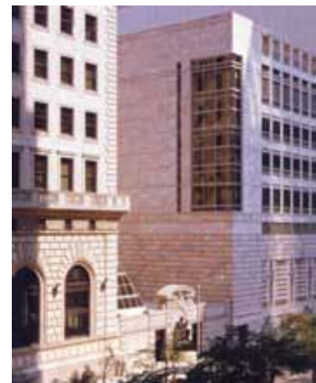
Stone veneer-faced precast panels clad the Federal Reserve Bank in Cleveland, Ohio.
