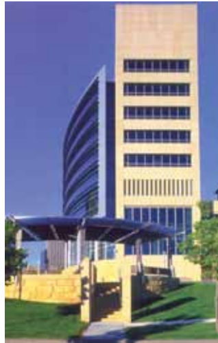
Precast cladding blended with the stone base of the Federal Reserve Bank in Minneapolis, Minn.
