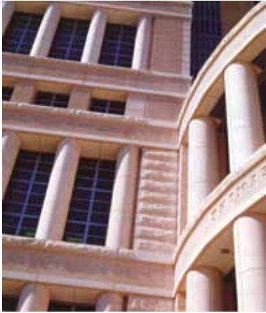
Close-up of rock-faced precast panels and lettering.
