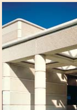
Form liner and sandblasted finish.
