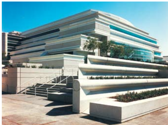
Fig. 3.3.16 Moscone Convention Center Esplanade Ballroom San Francisco, California; Architect: Gensler/DMJM, Associated Architects (joint venture).
