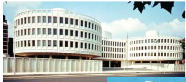
Fig. 1.2.4(a) Police Administration Building Philadelphia, Pennsylvania; Architect: Cubellis GBQC formerly Geddes Brecher Qualls Cunningham, Architects; Photos: Portland Cement Association.
