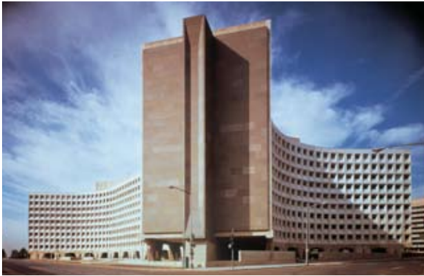
Fig. 1.2.5 U.S. Department of Housing and Urban Development Headquarters, Washington, D.C.; Architect: Marcel Breuer and Herbert Beckhard Design Architects; Nolen-Swinburne & Associates, Associate Architects; Photo: ©Images are courtesy of the Marcel Breuer papers, 1920-1986, in the Archives of American Art, Smithsonian Institution.
