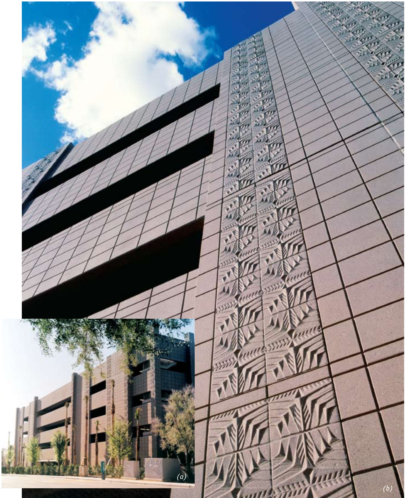
Fig. 3.5.17(a) & (b) Arizona Biltmore Parking Structure, Phoenix, Arizona; Architect: Nelsen Architects Inc.; Photos: Rod Eaves.
