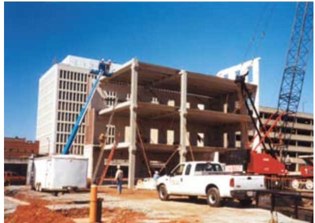
Precast Day 7 — Building begins taking shape.
