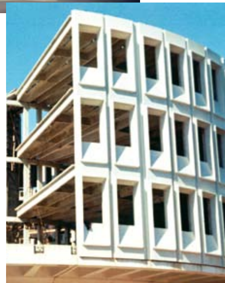
Fig. 1.2.4(b) Loadbearing wall construction.
