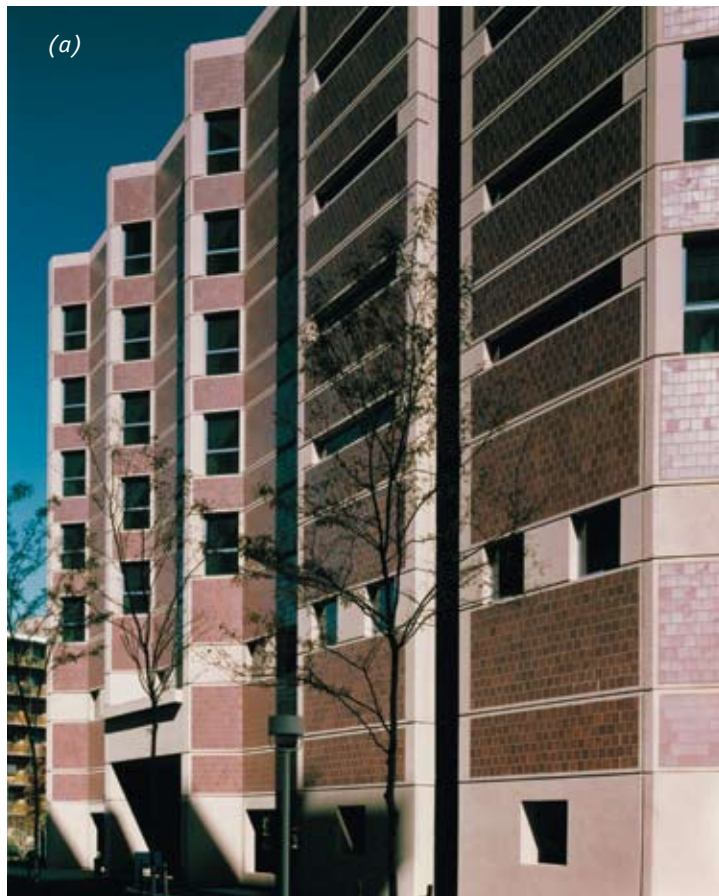
Fig. 3.5.62(a) & (b) Prospect Heights Care Center Hackensack, New Jersey; Architect: Herbert Beckhard Frank Richlan & Associates; Photos: Norman McGrath Photograph.
