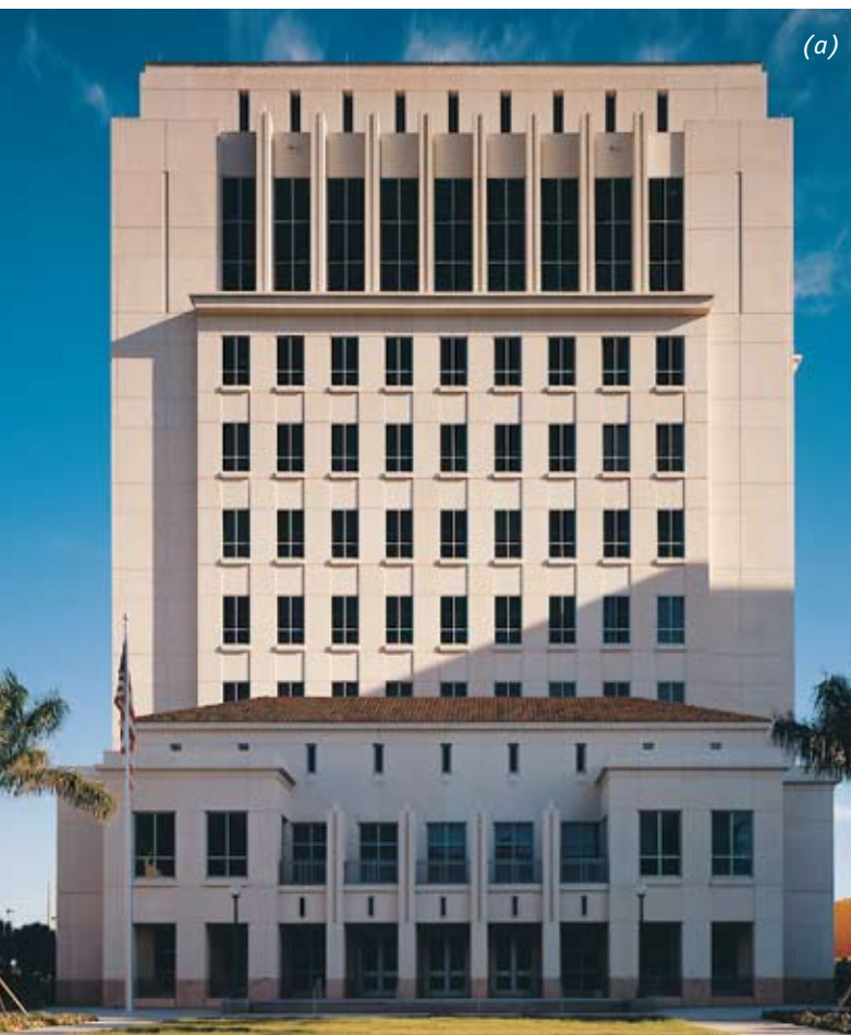
Fig. 2.6.1(a) & (b) Sarasota County Judicial Center, Sarasota, Florida; Architect: BMK Architects Inc. and HLM Design, Joint Venture Photos: Scott McDonald ©Hedrich Blessing.
