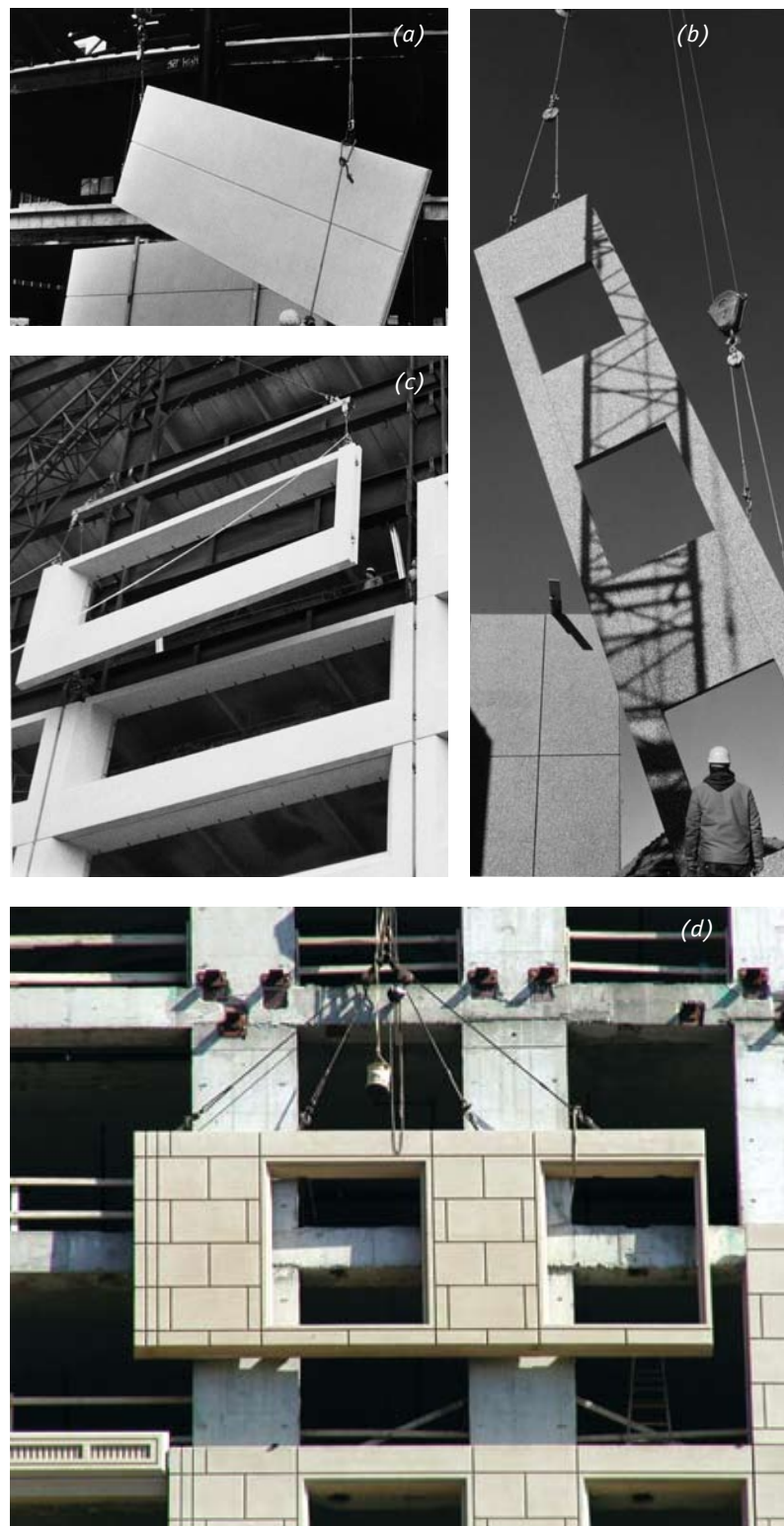
Fig. 4.2.18(a - d) Typical rigging arrangements.
