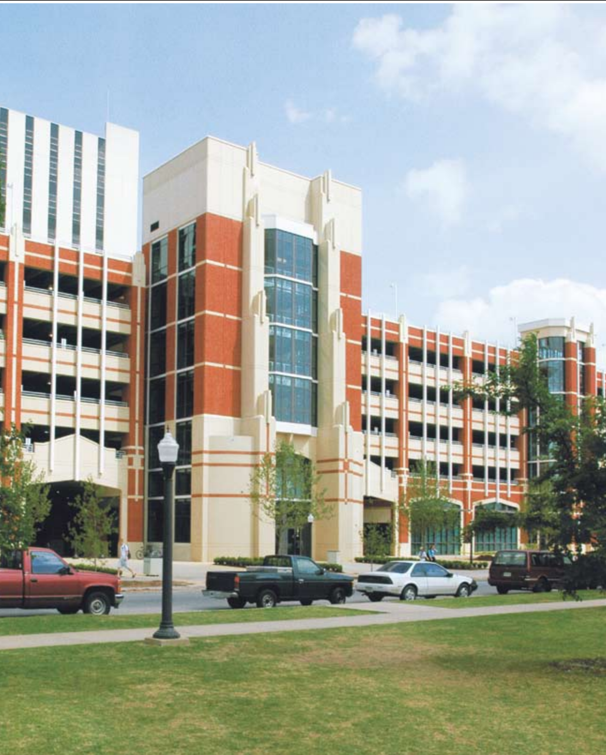
Asp Avenue Parking Facility Norman, Oklahoma; Architect: Frankfurt- Short-Bruza Associates.
