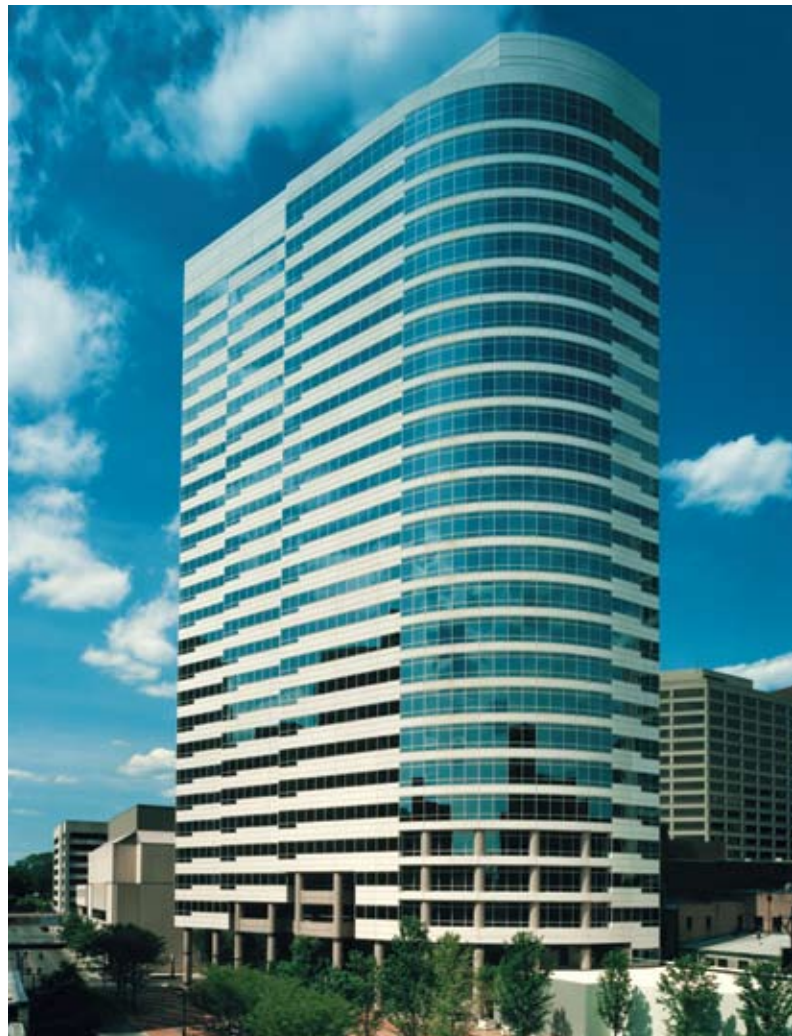
Fig. 2.4.3 Nashville City Center Nashville, Tennessee; Architect: The Stubbins Associates Inc.; Photo: Jonathan Hillyer.
