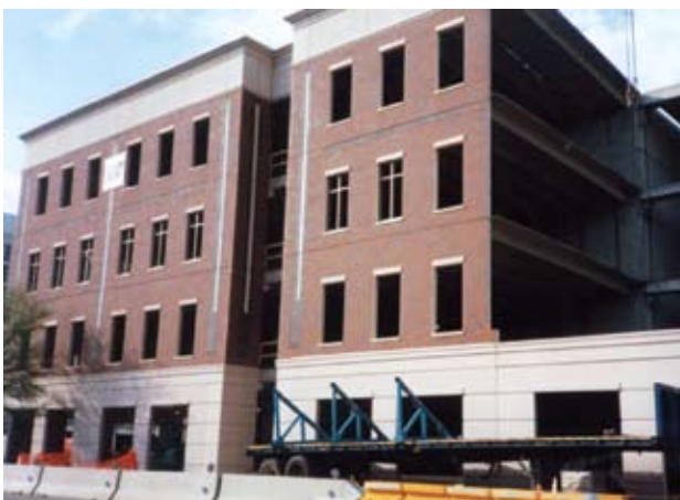
Precast Day 37 — Nearing completion.
