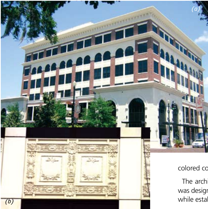
Fig. 3.5.19(a) & (b) 250 Park Avenue, Winter Park, Florida; Architect: Baker Barrios Architects Inc.; Design Consultant: Associated Consulting International; Photos: Phil Eschbach.
