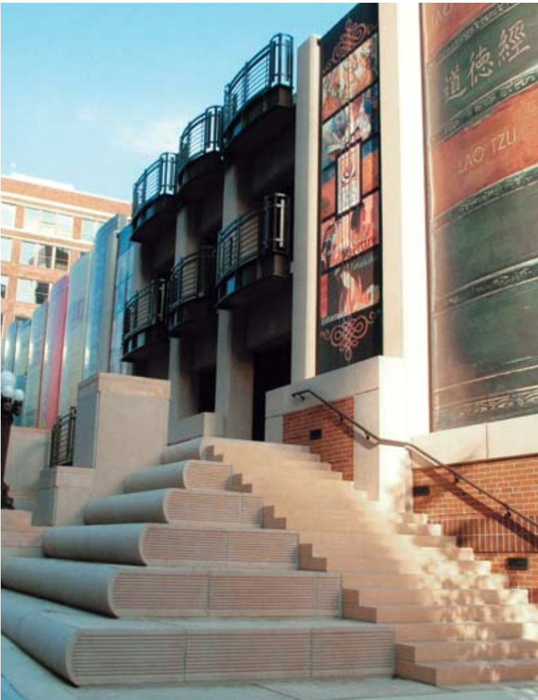
Fig. 1.3.11 Library District Parking Garage Kansas City, Missouri; Architect: BNIM and 360 Architecture (joint venture); Photo: BNIM/360.
