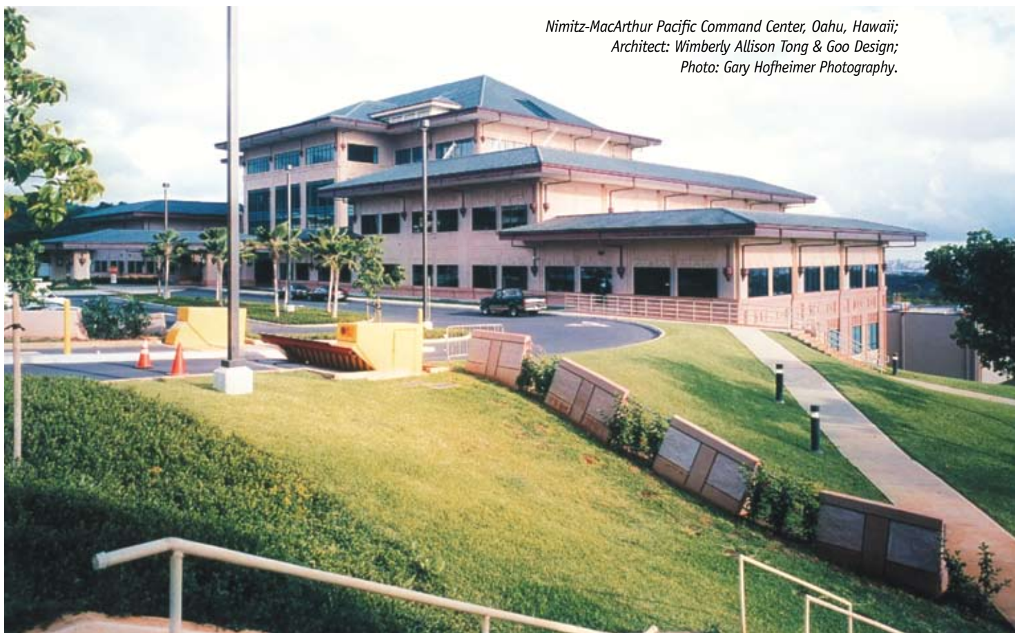
Fig. 5.6.7 Barriers to achieve standoff distance and limit vehicle access.
