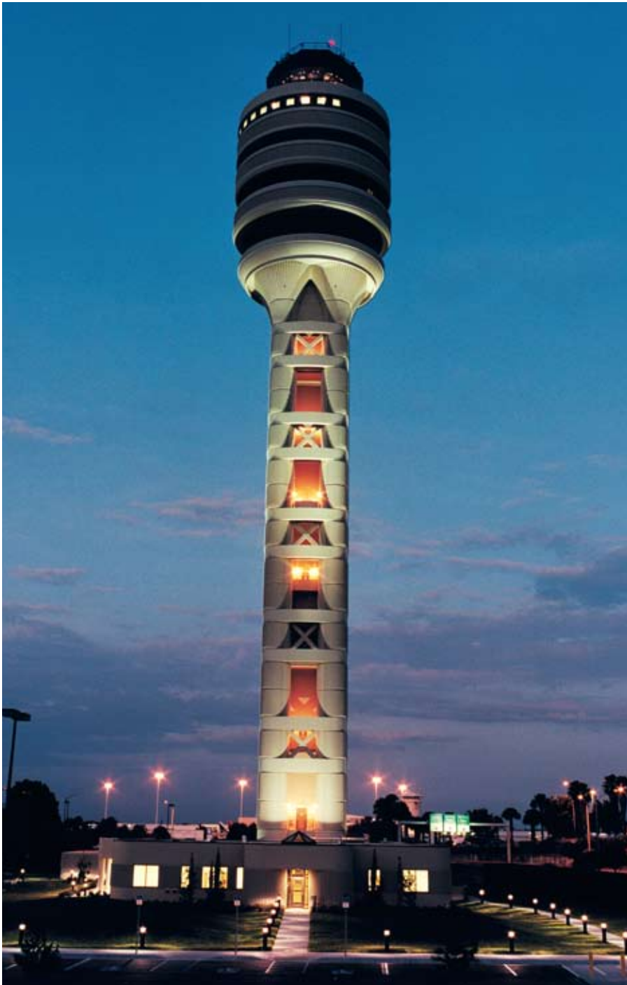
Fig. 1.3.6 Orlando International Air Traffic Control Tower, Orlando, Florida; Architect: URS Corporation (Radian International); Photo: Hensel Phelps Construction Co.
