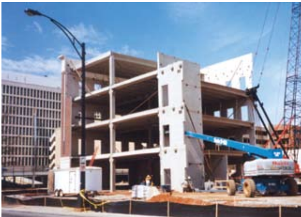
Precast Day 15 — Interior shear walls.
