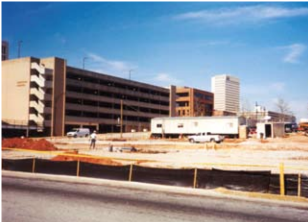
Precast Day 1 — Foundations ready, first piece arrives.
