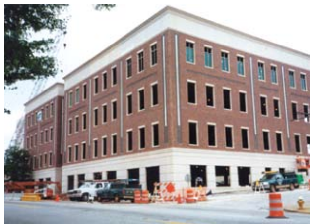
Precast Day 44 — Structurally and architecturally completed.
