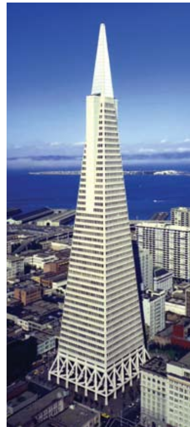
Fig. 1.2.6 TransAmerica Tower San Francisco, California; Architect: Johnson Fain and Pereira Associates (formerly William L. Pereira & Associates); Photo: Wayne Thom photographer.
