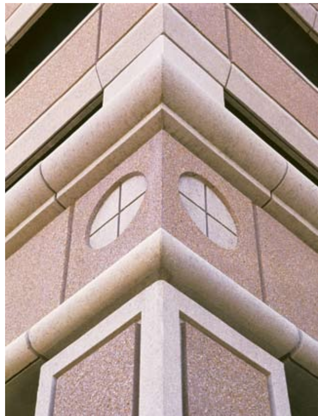
Fig. 3.5.10 Retarded and abrasive blasted finishes produced from the same concrete mix.
