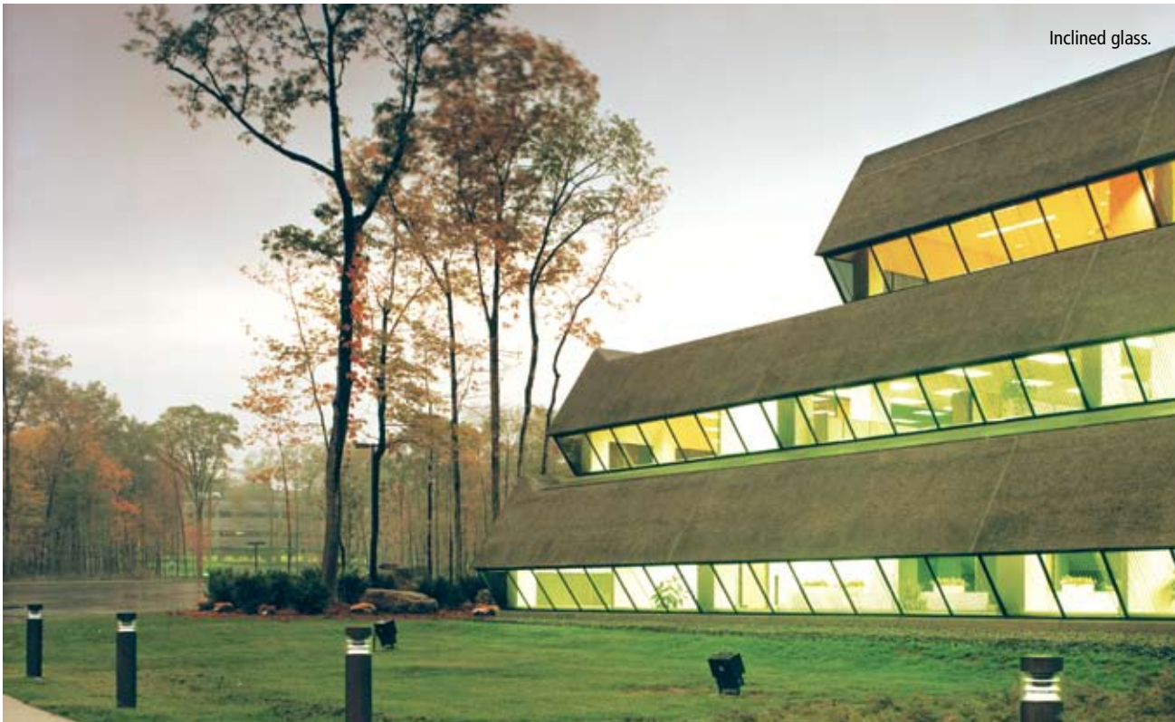
Fig. 5.3.13 Security Insurance Group Headquarters, Farmington, Connecticut; Architect: Russell Gibson von Dohlen; Photo: Steve Rosenthal.
