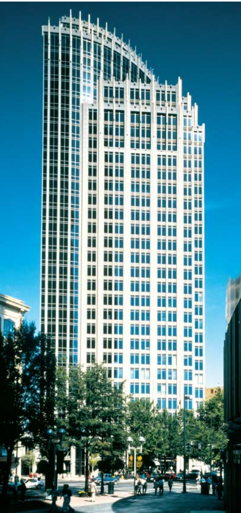
Fig. 1.2.3 IJL Financial Center, Charlotte, North Carolina; Architect: Smallwood, Reynolds, Stewart, Stewart & Associates, Inc.
