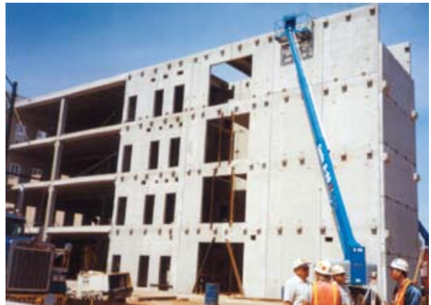
Precast Day 25 — Shear structure.
