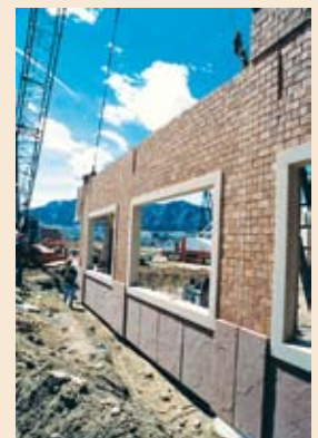
Thin brick, acid-etching and form liner.
