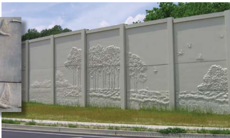
Maryland 216 Sound Barrier, Howard County, Md.; Designer/Engineer: JTE Civil Inc.; Photo: Creative Design Solutions.
