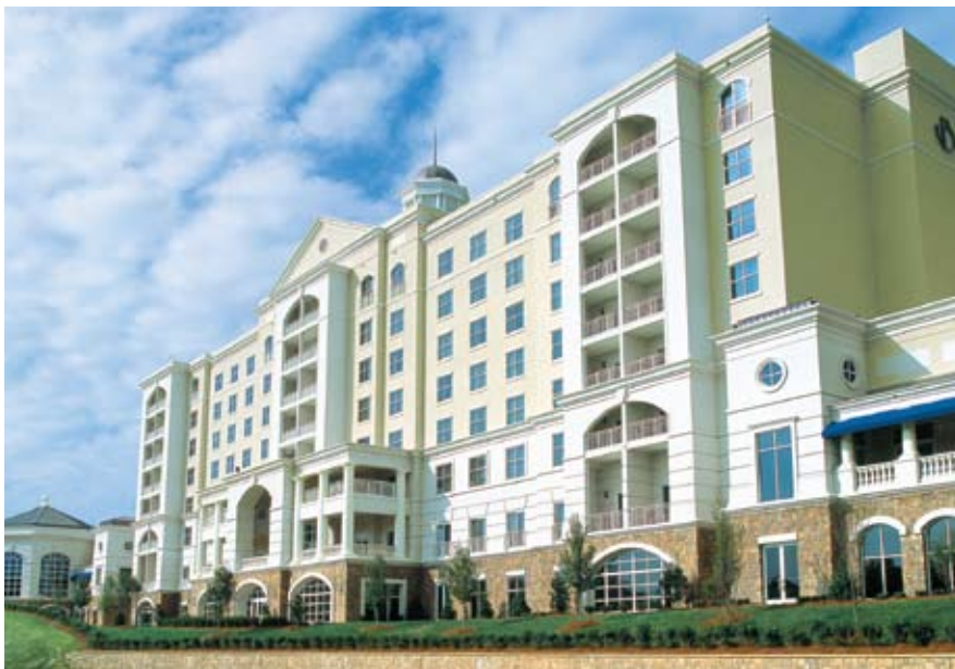
Ballantyne Resort Hotel, Charlotte, N.C.; Architect: LS3P Associates Ltd.
