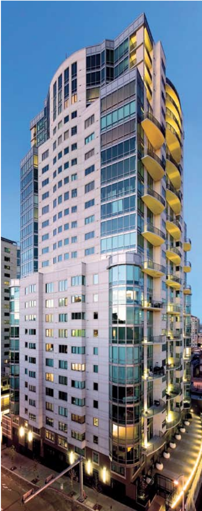
The Metropolitan, San Francisco, Calif.; Architect: Heller Manus; Architects and HKS.
