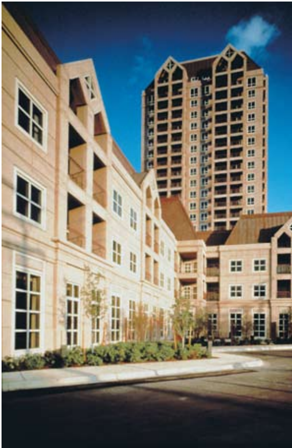
USAA Retirement Center, San Antonio, Tex.; Architect: HKS Inc.
