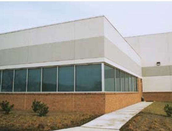
Federal Express, Crofton, Md.; Architect: Morgan Glick & Associates.
