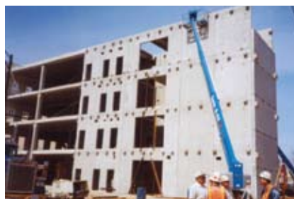
Day 25 — Shear structure.
