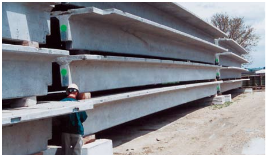
In the yard, the auditor ensures that components are stored properly. These double tees have been painted with green dots to indicate that they have passed the precaster's quality control check.
