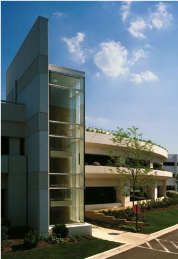
Resurrection Medical Center Southeast Parking Structure, Chicago, Ill.; Architect: Loeb Schlossman & Hackl.
