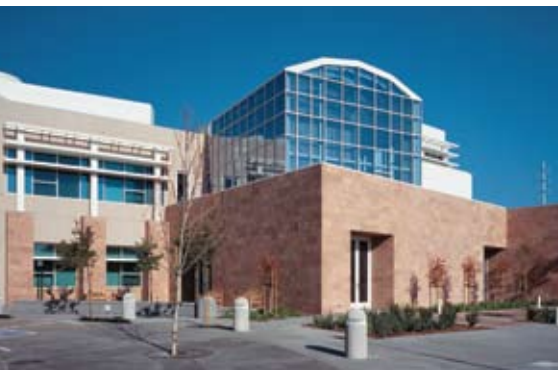
Arizona red sandstone, 1 1/4 in. to 1 3/4 in. thick, was anchored to 4-in.-thick concrete panels for the Sacramento Municipal Utility District's Customer Service Center, Sacramento, Calif.; Architect: Williams + Paddon Architects & Planners/Inc.
