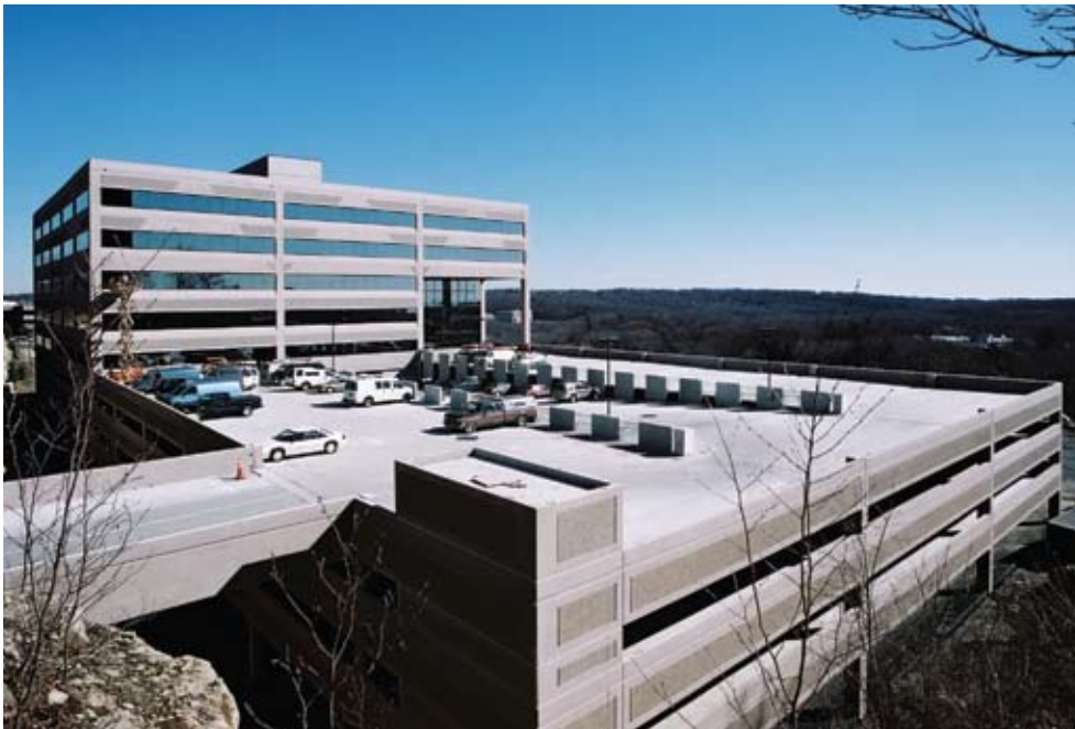
Enterprise IV Corporate Center, Bridgeport, Conn.; Architect: Kasper Group Inc.; Photo: Blakeslee Prestress.
