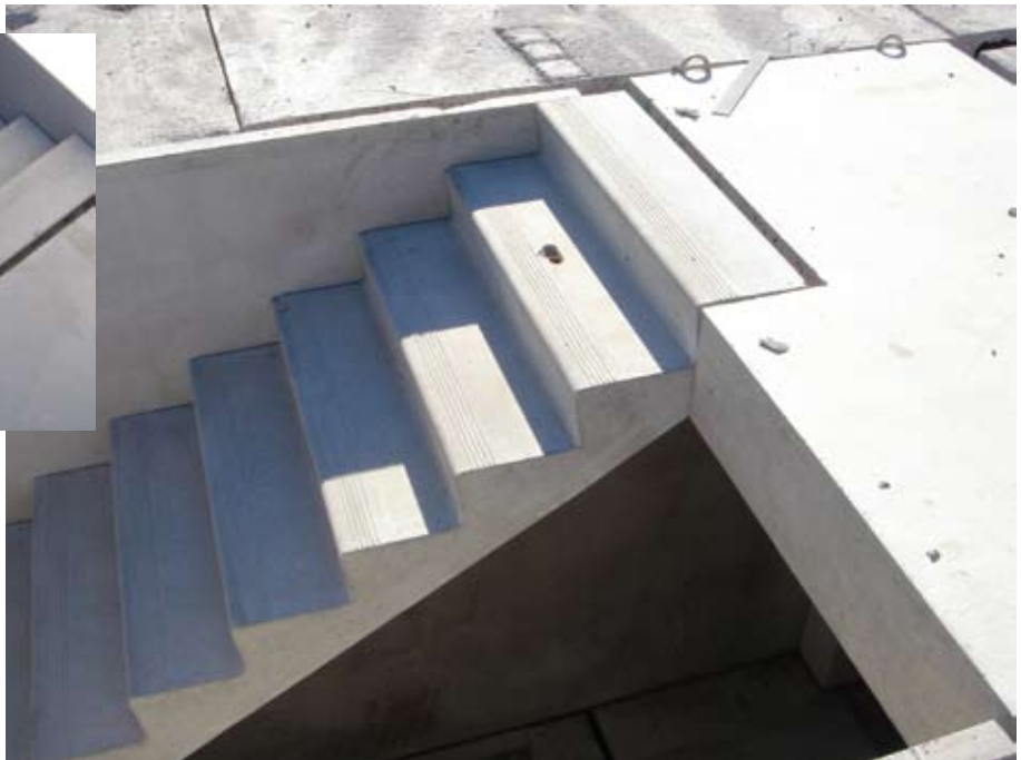
Stair run supported by precast concrete landing.
