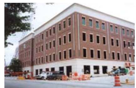
Day 44 — Structurally and architecturally dry.
