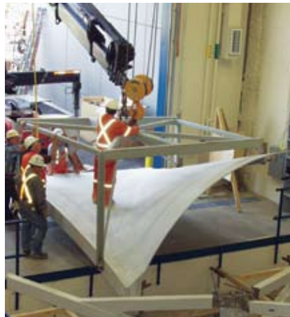
Installation of the prototype canopy at the University of Calgary's Centre for Innovative Technology. Photo: courtesy LaFarge.
