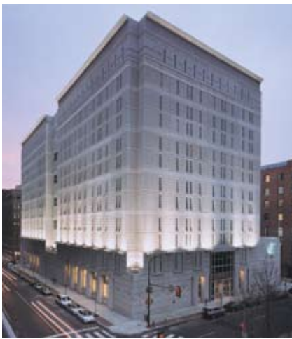
Federal Metropolitan Detention Center, Philadelphia, Pa.; Architect: Ewing Cole Cherry Brott; Photo: Jeffrey Totaro.
