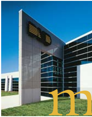
Digital Monitoring Products Inc., Springfield, Mo.; Architect: Sapp Design Associates Architects P.C.
