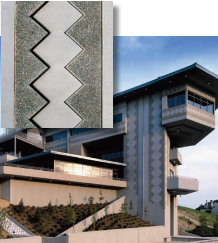
Utoy Creek Water Reclamation Center, Atlanta, Ga.; Architect: ; Photos: .
