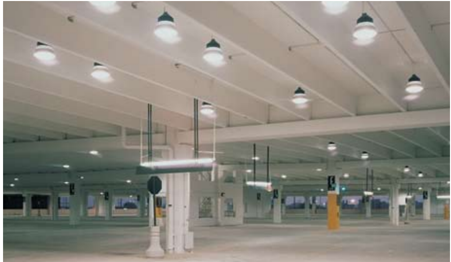
The three parking structures for the Shops at Willow Bend Mall in Plano, Tex., provide a light, bright interior. JPRA Architects Inc., Farmington Hills, Mich. Photo: J. Bendist Photographic/Dallas.
