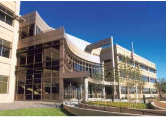
The United States Department of Transportation facility in Lakewood, Colo., used an all-precast concrete structure to help it achieve LEED Silver Certification. Design Architect: Oz Architecture; Architect/engineer: Opus Architects & Engineers Inc.; Photo: Oz Architecture.
