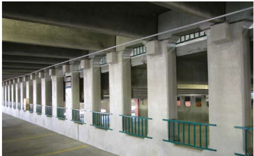
Union Plaza Transit Terminal and Parking Garage, El Paso, Tex. The use of an all-precast concrete structure, including double tees, beams, columns, and shear walls speeded construction and maximized interior layout space.
