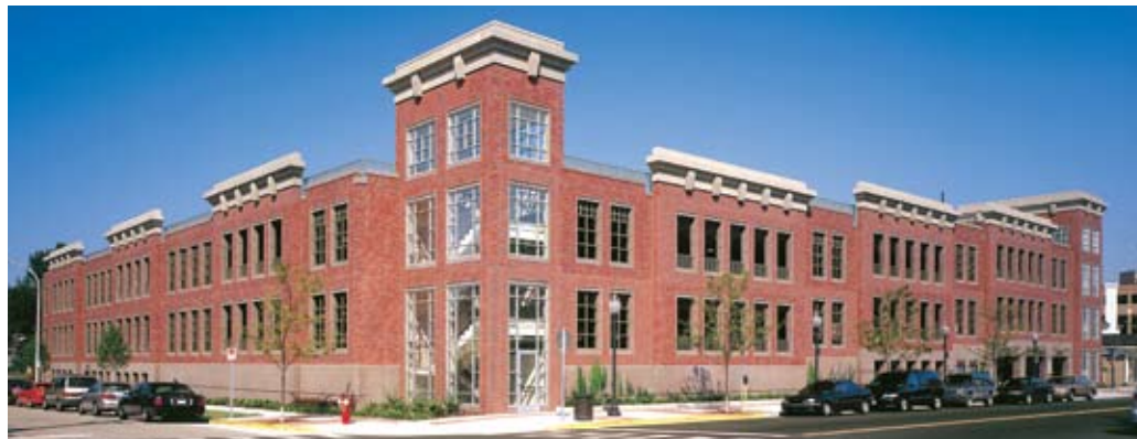
Fifth and Lafayette Parking Structure, Royal Oak, Mich.
