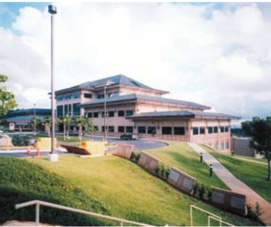
Nimitz-MacArthur Pacific Command Center, Oahu, Hawaii; Architect: Wimberly Allison Tong & Goo Design; Photo: Gary Hofheimer Photography.
