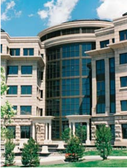
Starz Encore Headquarters (total precast), Englewood, Colo.; Architect: Barber Architecture; Photo: David Cornwell Photography.
