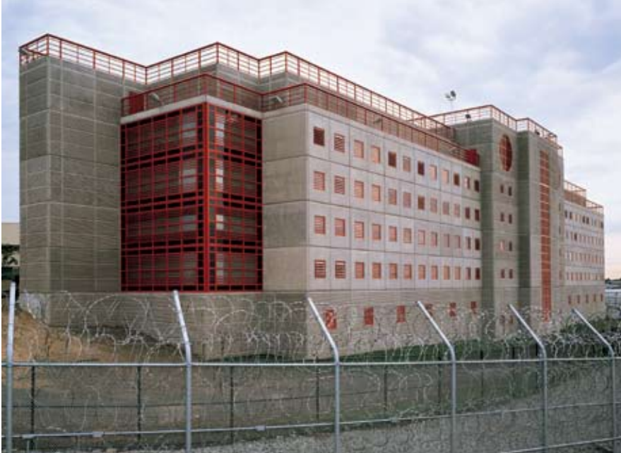
George R. Vierno Center Addition, Rikers Island, New York; Architect: STV/Silver & Ziskind; Photo: S. Barker.
