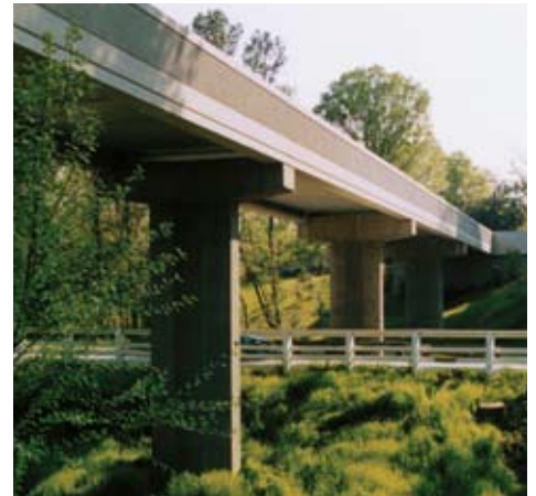
Colonial Williamsburg Bridge To The Past, Williamsburg, Va.; Architect: Carlton Abbott & Partners PC.
