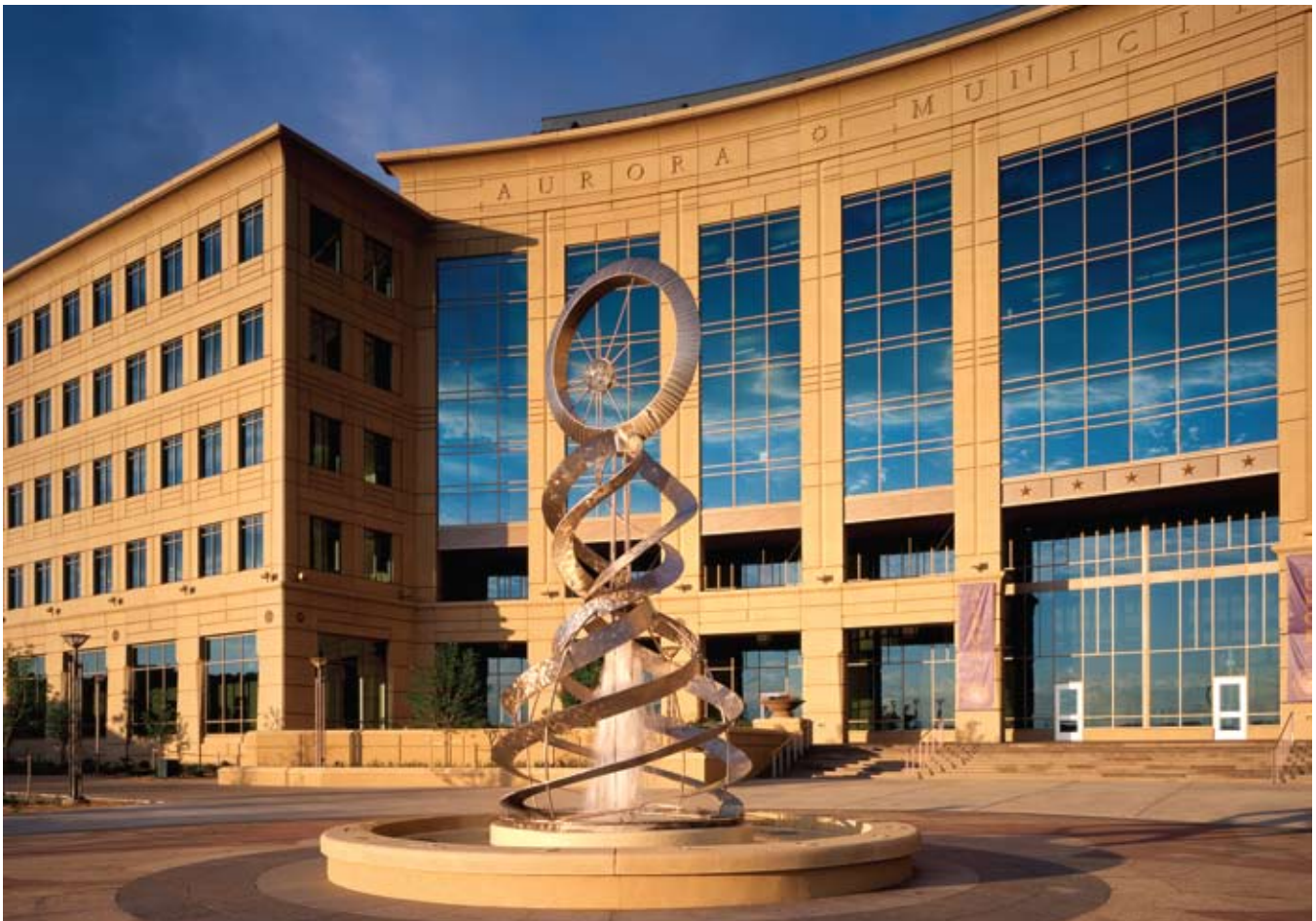
Aurora Municipal Center, Aurora, Colo.; Architect: Barber Architecture.
