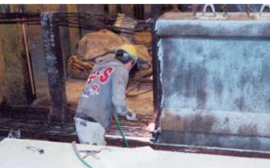
For this bridge girder being manufactured, cutting torches are being used to detension the strand.
