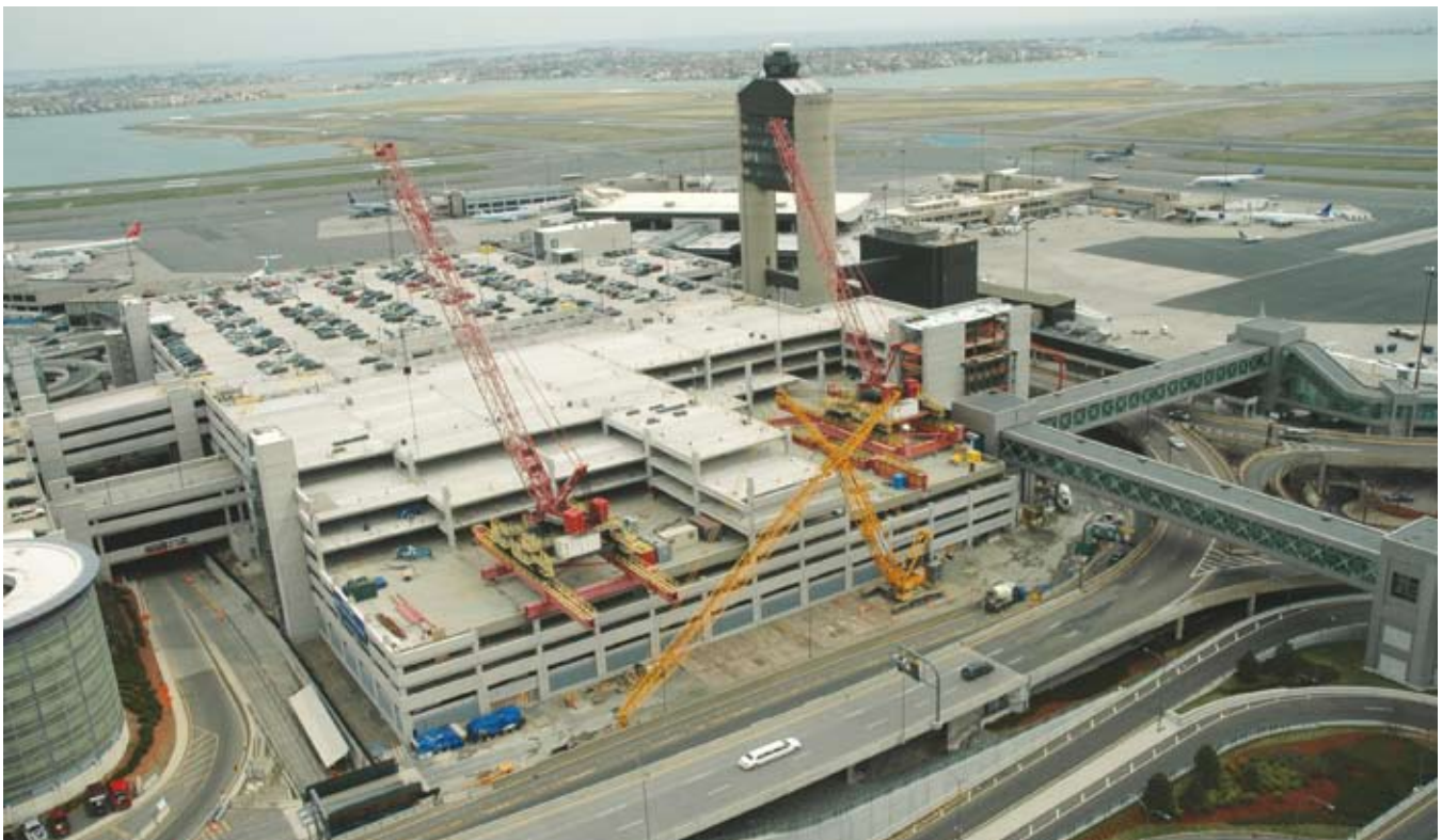
Logan International Airport Central Parking Garage Expansion, Boston, Mass.; Architect: TAMS/Fennick/McCredie Architecture Ltd.; Photo: Blakeslee Prestress Inc.
