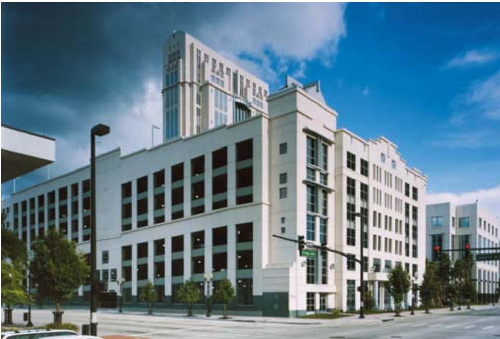
Orlando County Courthouse Parking Structure Expansion, Orlando, Fla.; Architect: Burke, Hogue & Mills Associates Inc.
