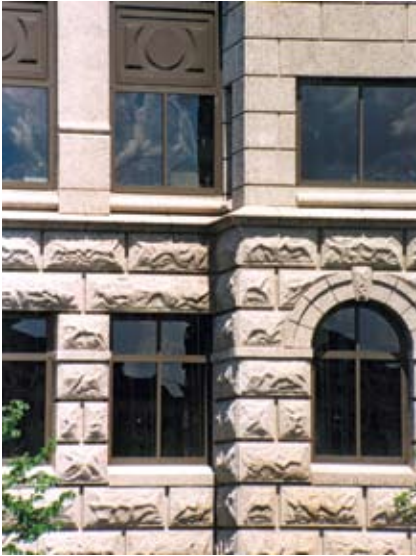
The Starz Encore building in Denver, Colo., features several finishes, including a cut-stone style created with a formliner made from actual stone samples.
