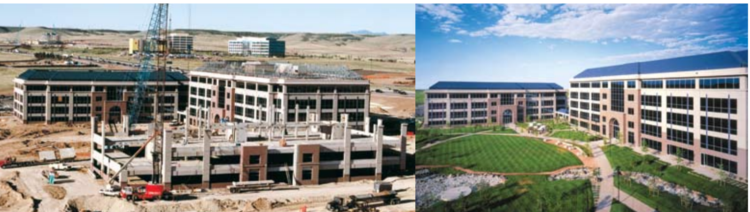
CH2M Hill World Headquarters, Englewood, Colo.; Architect: Barber Architecture, Denver, Colo.; Photos: Rocky Mountain Prestress.
