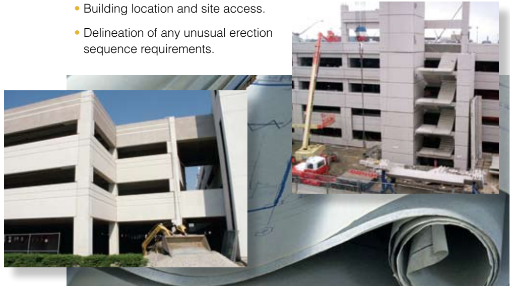
Logan International Airport Central Parking Garage Expansion, Boston; Architect; TAMS/Fennick/McCredie Architecture Ltd.; Photo: Blakeslee Prestress Inc. (top right), ©PhotoDisc (bottom right).
