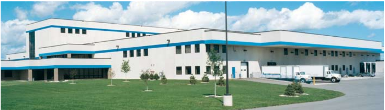
Gannett Newspapers, Appleton, Wis.; Architect: McMahon Associates.
