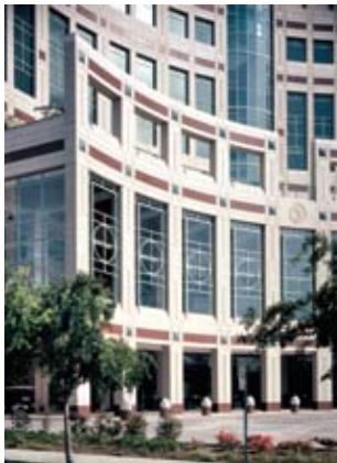
Panels on the Shriners Hospital for Crippled Children, Sacramento, Calif., are 6 in. thick and have a horizontal band of 1 1/4 in. granite attached with one anchor per 2 ft 2 . Architects: Odell Associates; and Associate Architect: HDR.
