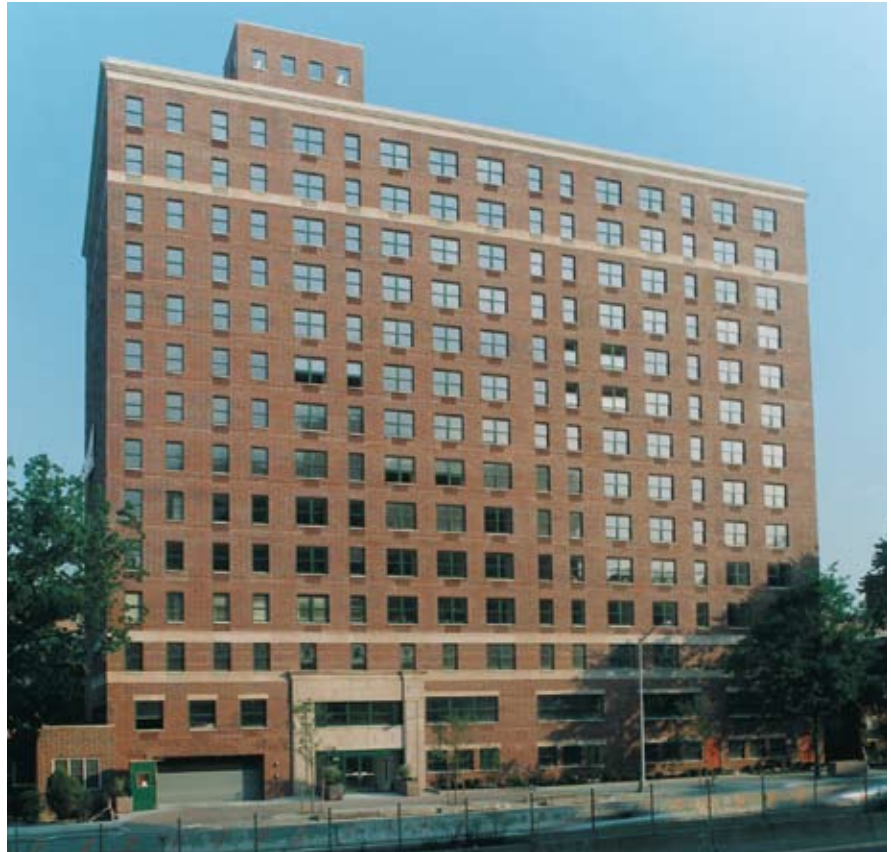
Senior Quarters at Riverdale, Bronx, N.Y.; Architect: Architects Design Group.
