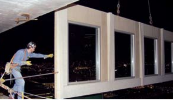
This typical panel contains four preglazed windows for a 42-story building. Each panel has four tones of color created by heavy and light sandblasting of two colors of precast concrete.
