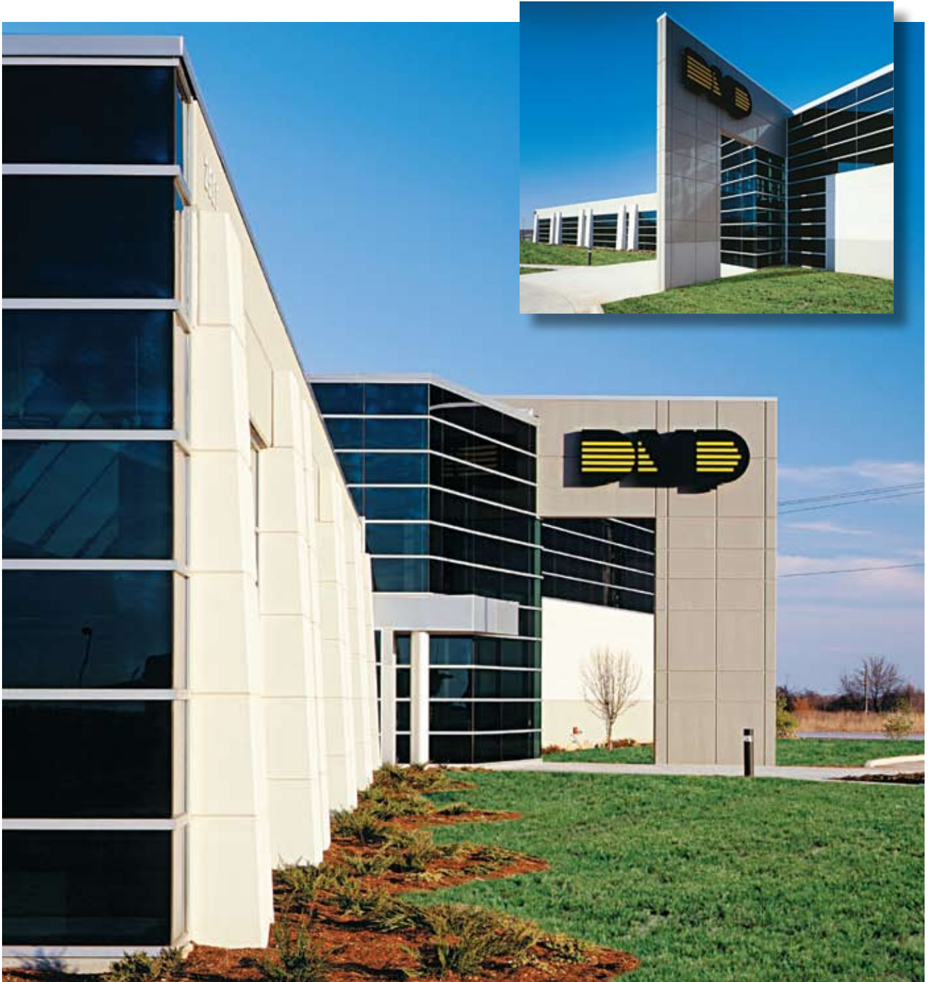
Digital Monitoring Products Inc., Springfield, Mo.; Architect: Sapp Design Associates Architects P.C.
