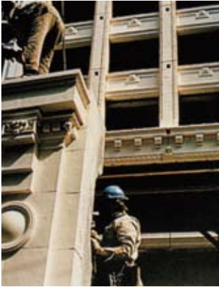
Built in 1906, the architectural landmark 88 Kearney St. in San Francisco had its terra cotta removed and reassembled on precast panels for an all-new structure of taller height. Architect: Skidmore, Owings & Merrill; Photo: Skidmore, Owings & Merrill.
