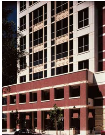
One-in.-thick brick cladding on 5-in.-thick concrete panels was used on the first three floors of the Sacramento County System and Data Processing Building in Sacramento, Calif. Terracotta medallions were placed on spandrels and column covers. Architect: HDR Architecture Inc. formerly Ehrlich-Rominger; Photos: HDR Architecture Inc.
