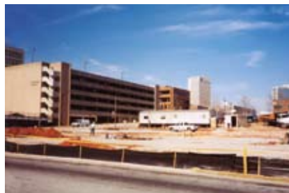
Day 1 — Foundation ready.
