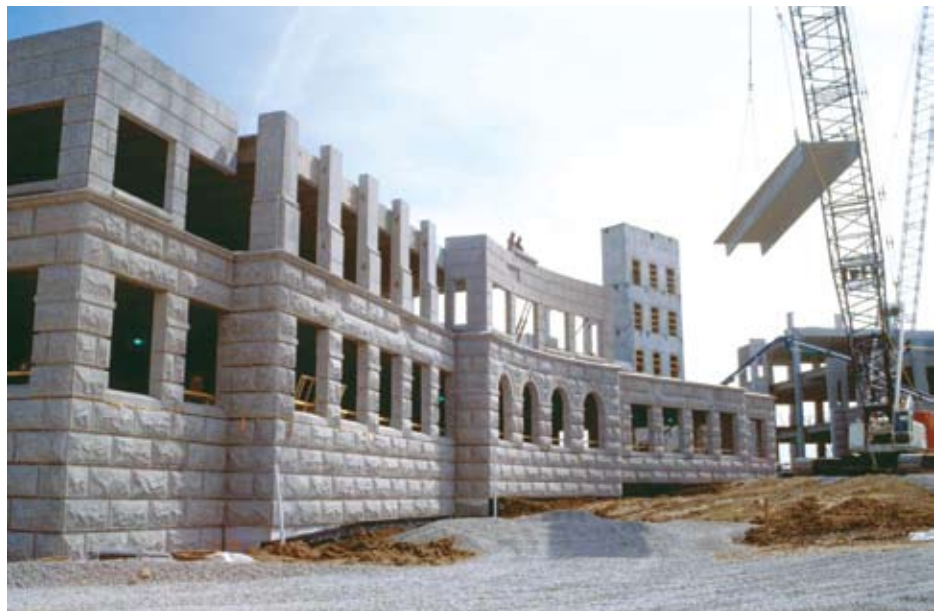
The all-precast concrete structural system includes double tees, inverted tee beams, shear walls, and loadbearing precast walls. The system is a common approach to design in the Rocky Mountain region.
