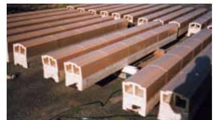
One-in.-thick brick cladding on 5-in.-thick concrete panels was used on the first three floors of the Sacramento County System and Data Processing Building in Sacramento, Calif. Terracotta medallions were placed on spandrels and column covers. Architect: HDR Architecture Inc. formerly Ehrlich-Rominger; Photos: HDR Architecture Inc.
