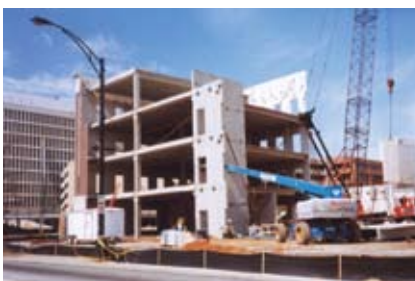
Day 15 — Interior shear walls.
