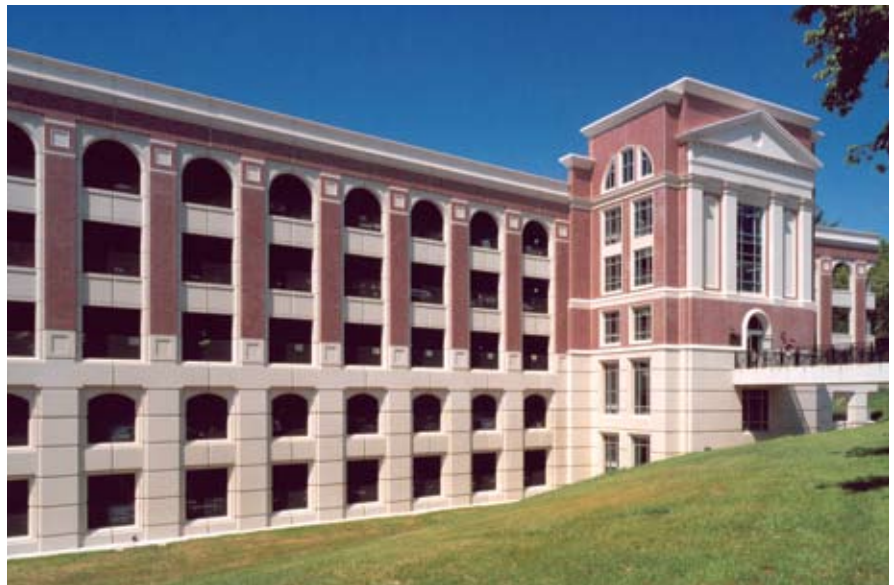
Hull Street Parking Structure, Athens, Ga.; Architect: Smallwood, Reynolds, Stewart, Stewart & Associates Inc.; Photo: Jim Roof.
