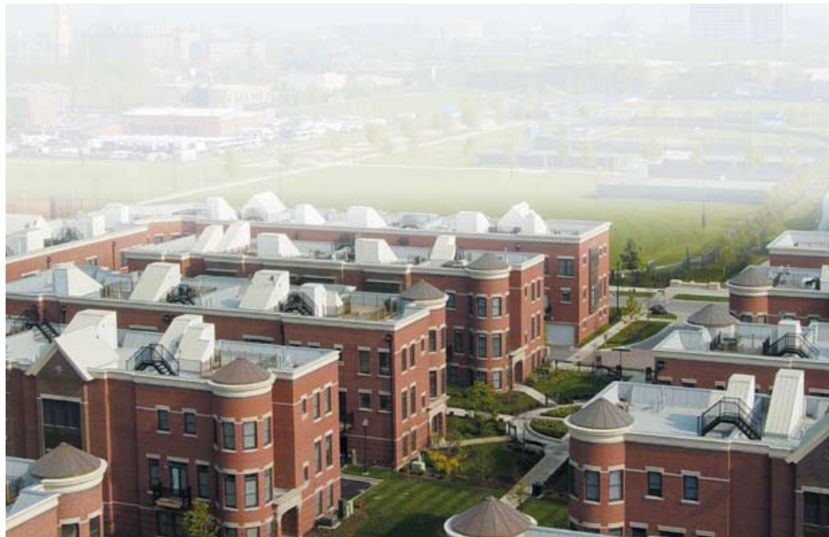
University Village, Chicago, Ill.; Architect: FitzGerald Associates Architects; Photo: The Spancrete Group.
