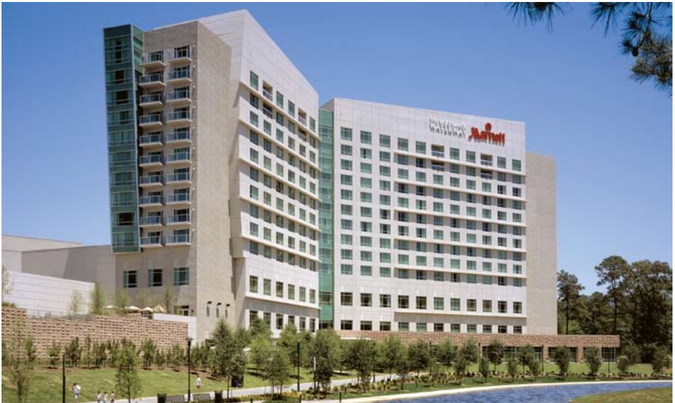
Woodlands Waterway Marriott Hotel & Conference Center, The Woodlands, Tex.; Architect: Gensler.
