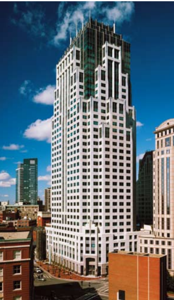
State Street Financial Center, Boston, Mass.; Architect: Jung/Brannen Associates Inc., Boston, Mass.; Photo: Peter Vanderwarker.
