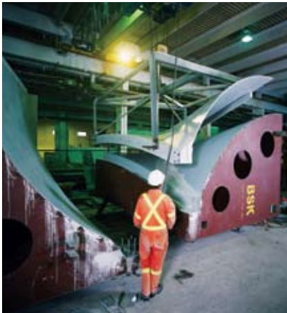
Demolding of the precast concrete canopy element. Photo: © Tucker Photo.
