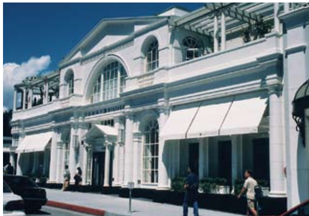
Tommy Hilfiger Retail Incorporated, Beverly Hills, Calif.; Architect: Allan Greenberg, Architect; Photo: David Rath.
