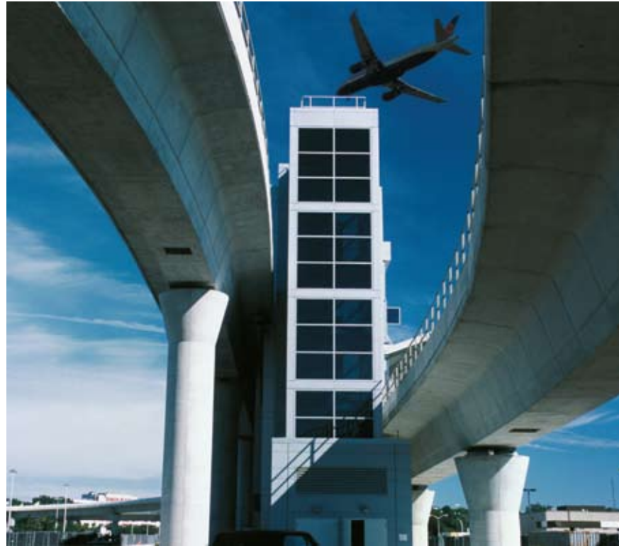
AirTrain Light Rail System, Queens, N.Y.
