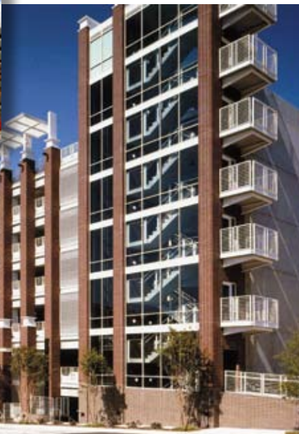
South Spring Street Garage, Greenville, S.C.; Architect: Craig Gaulden Davis, Greenville, S.C.; Consulting Architect: LS3P Associates Ltd., Charlotte, N.C.
