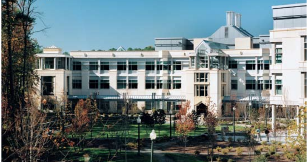
Levine Science Research Center at Duke University, Durham, N.C.; Architect: Payette Associates Inc.; Photo: Brian Vanden Brink.
