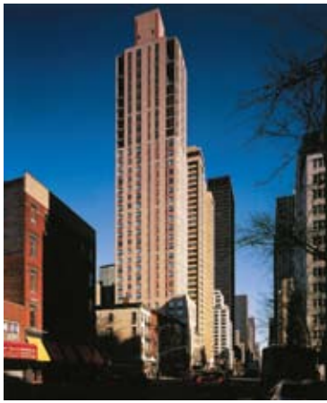
Third Avenue Marriott ExecuStay, New York City; Architect: H. Thomas O'Hara Architects.
