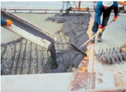
Self-consolidating concrete flows quickly into place to fill every nook, leaving no voids and producing a smooth, densely packed finish.
