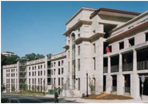
Emory University Parking Structure, Atlanta, Ga.; Architect: Thompson, Ventulett, Stainback and Associates Architects (TVS); Photo: Brian Cassel/TVS.
