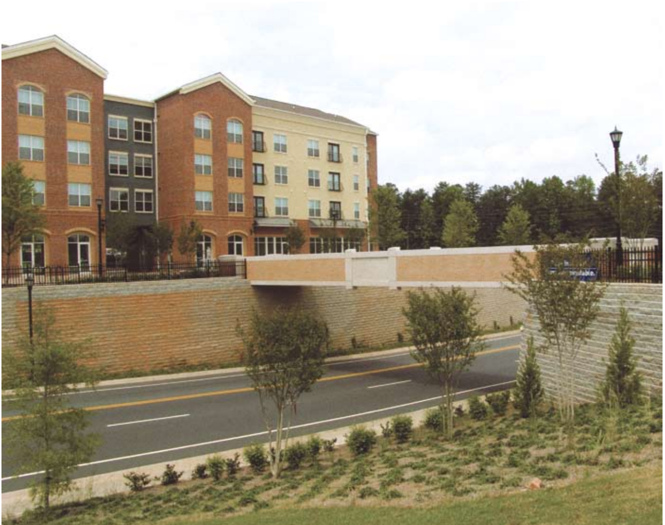
Kennesaw State University Phase II Pedestrian Bridge, Kennesaw, Ga.; Architect: Niles Bolton Associates.
