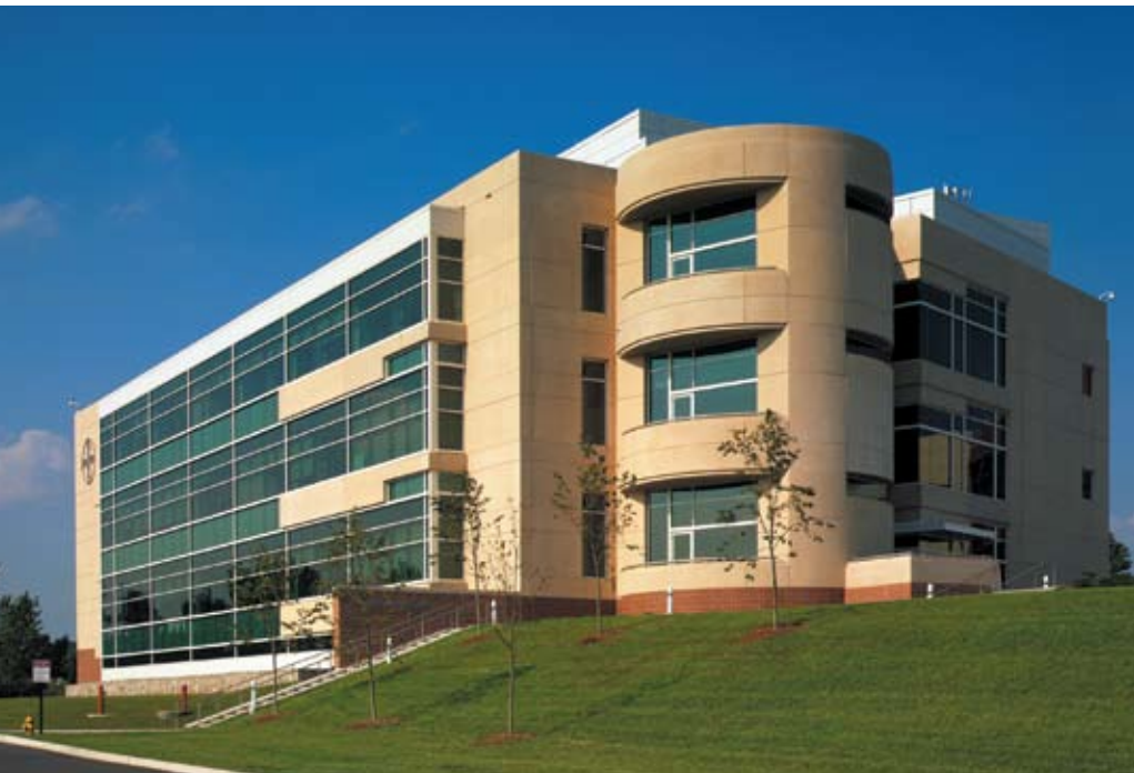
Bayer Corp. B27 Building, West Haven, Conn.; Architect: Flad & Associates; Photo: ©Burne Photo Imaging Inc.
