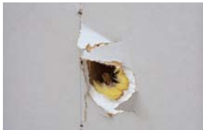
In test one, the 2 x 4 went through this vinyl sided, wood-frame wall panel like a hot knife through butter. Notice the entry, and the exit holes. Not only are they clean holes, but it didn't even slow the projectile down.
