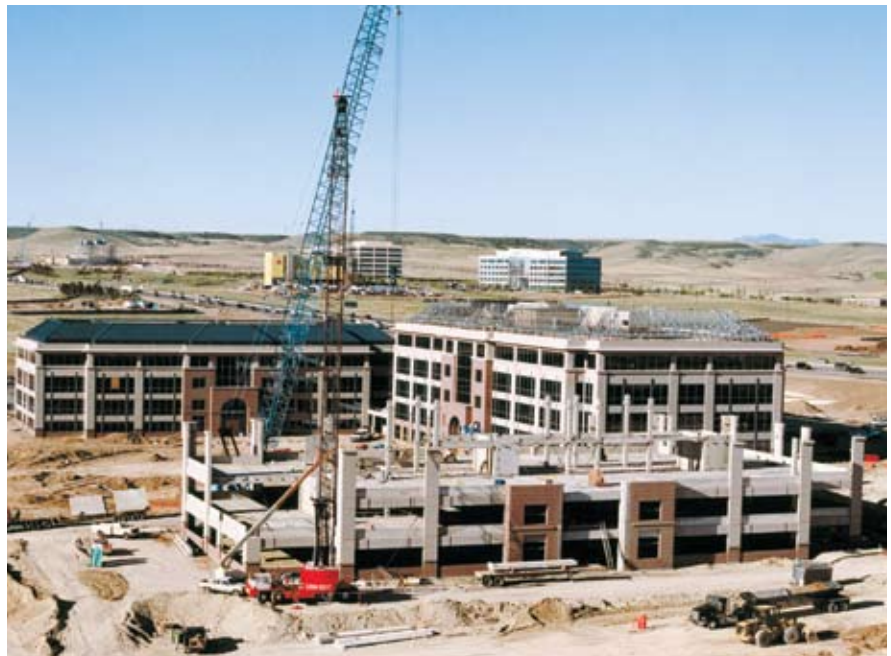
All three structures in the Starz Encore complex in Denver, Colo., feature total precast structural systems and were designed, fabricated, and erected in 11 months.
