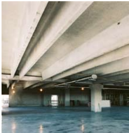
The Enterprise IV project features double tees as flooring, which create large, open floor plans that add flexibility for tenants.
