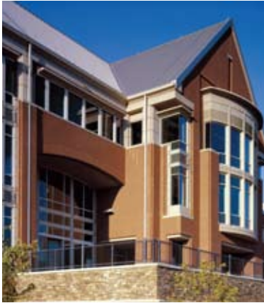
Merrill Lynch Hopewell Campus, Pennington, N.J.; Architect: Thompson, Ventulett, Stainback & Associates (TVS&A); Photo: TVS&A.
