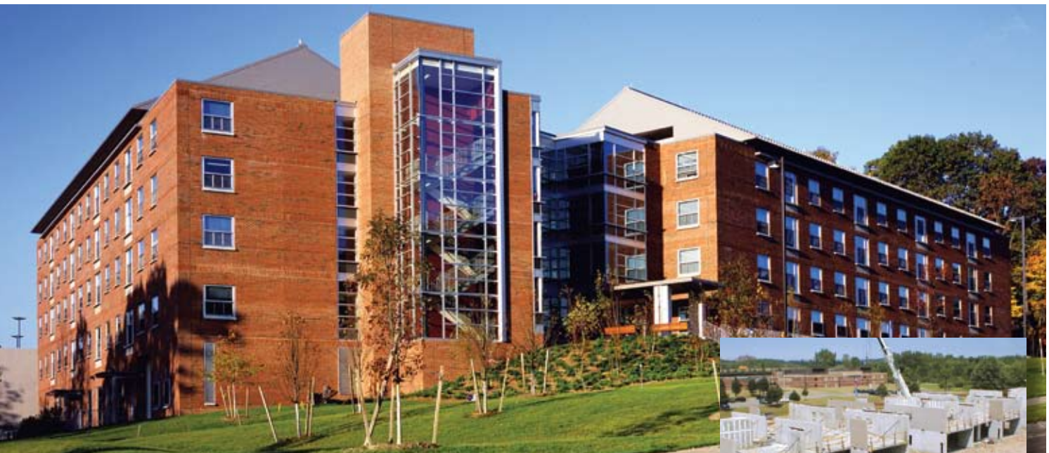
Western Connecticut State University Dormitory, Danbury, Conn.; Architect: Herbert S. Newman & Partners PC; Photos: Blakeslee Prestress Co.
