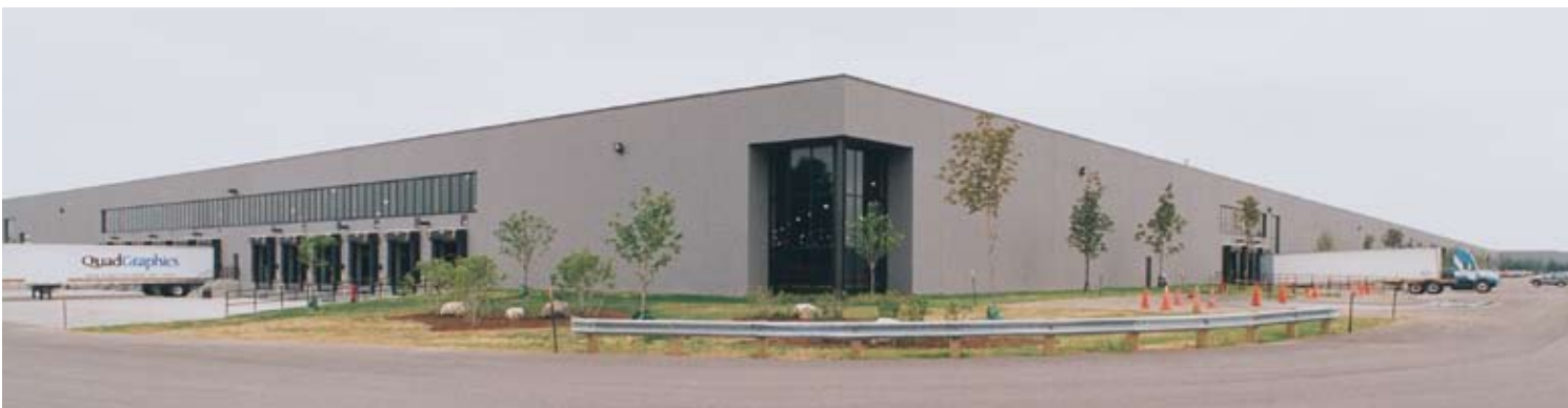
Quad Graphics, Wis.; Architect: Wheeler-Kearns Architects; Photo: William Kildow.
