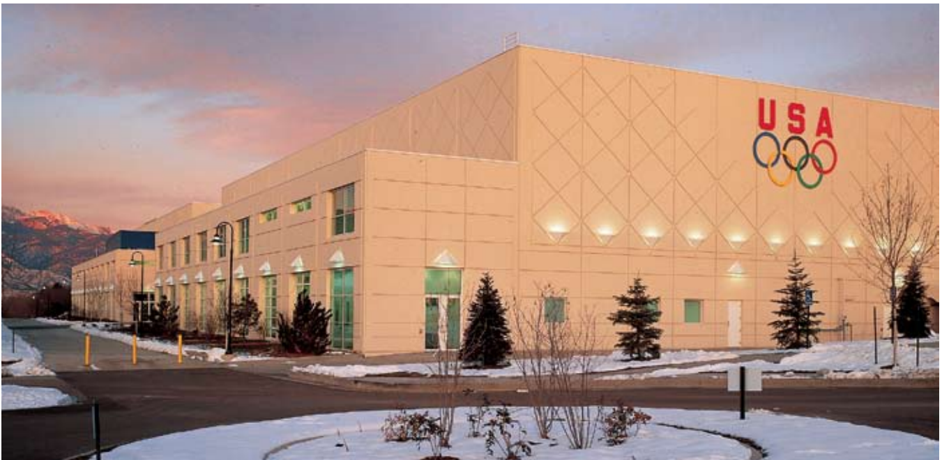
U.S. Olympic Center, Colorado Springs, Colo.; Photo: John Miller, Hedrich Blessing.
