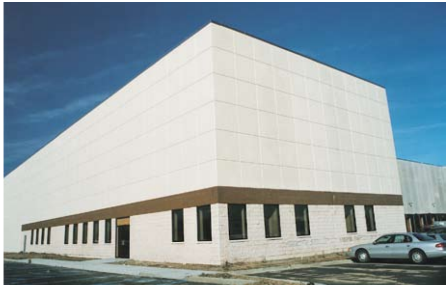
Lily Popcorn Co., Bethpage, N.Y.; Architect: Billow & Goldberg Associates.
