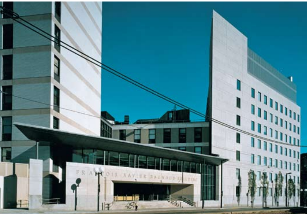
Francois-Xavier Bagnoud Building, Harvard School of Public Health, Boston, Mass.; Architect: Payette Associates Inc.
