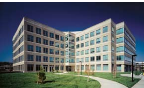
GFRC with horizontal striations relate the Pleasanton Corporate Campus buildings to the hills, creating the texture and shadow pattern HOK/SF Inc. Architects were looking for. Photo: HOK/SF Inc.
