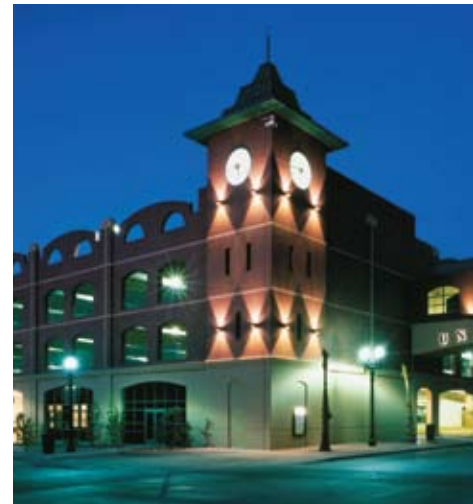
Union Plaza Transit Terminal and Parking Garage, El Paso, Tex.; Architect: Synthesis Architecture Inc.
