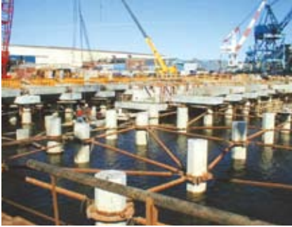
Bath Iron Works Land Level Transfer Facility, Bath, Maine.
