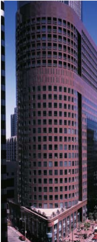
388 Market Street building in San Francisco, Calif., is clad with 1 1/4 in. (3 cm) granite anchored to precast concrete. Architect: Skidmore, Owings & Merrill; Photo: Skidmore, Owings & Merrill San Francisco.
