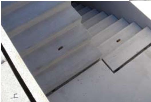
Velocity Multifamily Residential Condos, Hoboken, N.J.; Architect: Equus Design Group; Photos: Oldcastle.
