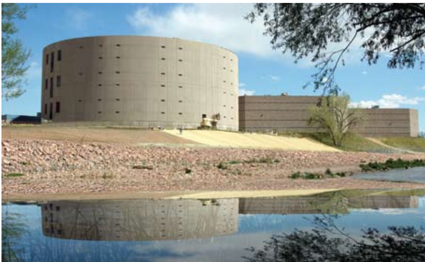
El Paso County Jail, Colorado Springs, Colo.; Architect: CSNA Architects.
