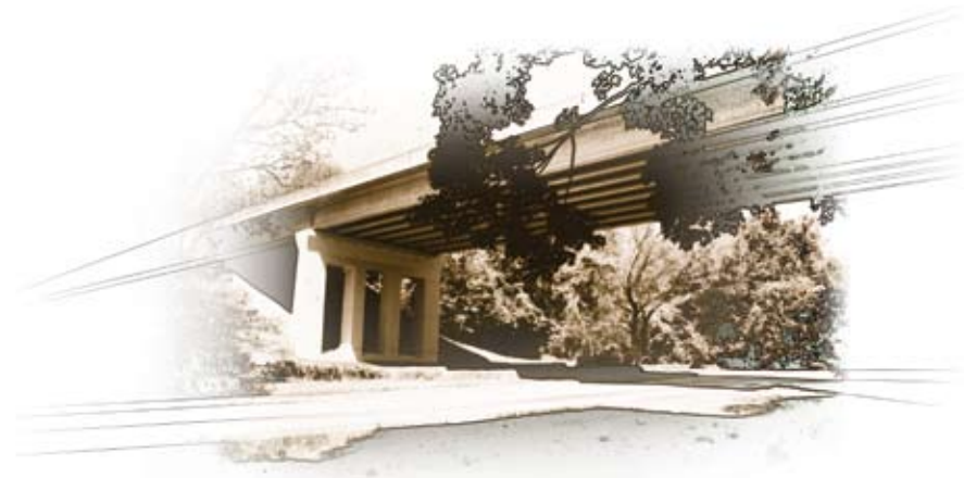
Walnut Lane Memorial Bridge; Philadelphia, Pa.
