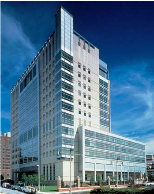
Abraham Pediatric Research Center, Children's Hospital of Philadelphia, Pa.; Architect: Ellenzweig Associates; Photo: Tom Crane.
