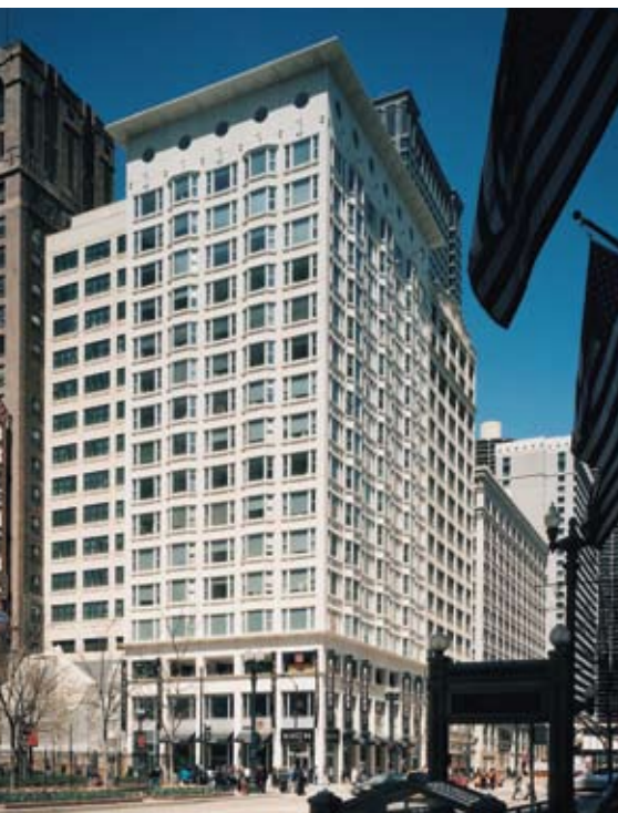
Located in downtown Chicago, Ill., the new residence hall for the School of the Art Institute is clad in GFRP panels, which emulate the look of the Windy City's historic buildings finished in terra cotta. The dormitory is composed of two connected buildings and a rear link. Architect: Booth Hansen Associates Inc., Chicago; Photo: ©Brian Fritz Photography.
