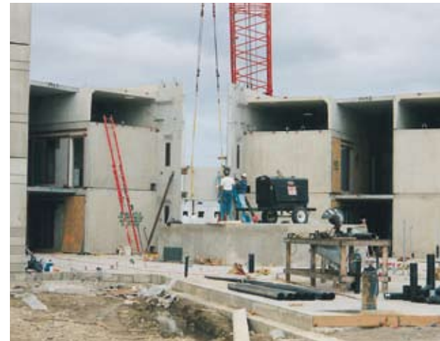
Two converging wings of Special Housing under construction expose the precast components of the building; stacked modular cells, hollow-core slab corridors, plenums, and insulated wall panels.
