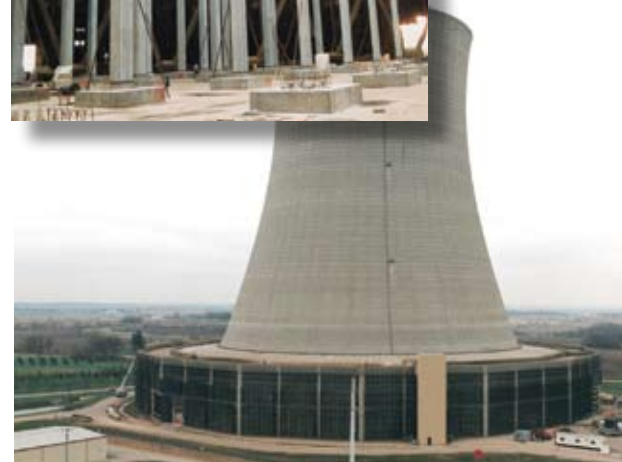
Commonwealth Edison Cooling Tower, Bryon, Ill.
