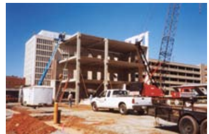
Day 7 — Building begins taking shape.
