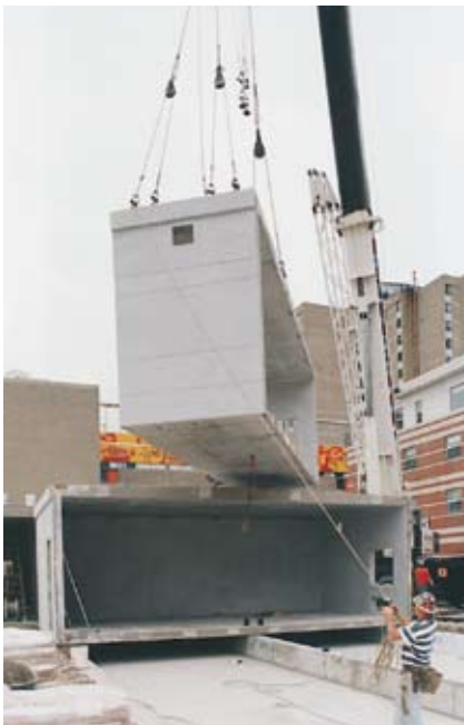
A crane hoists one of the 30-ft modules into place on the concrete foundation. The modules were delivered at night under a police escort because of daytime congestion in the area.
