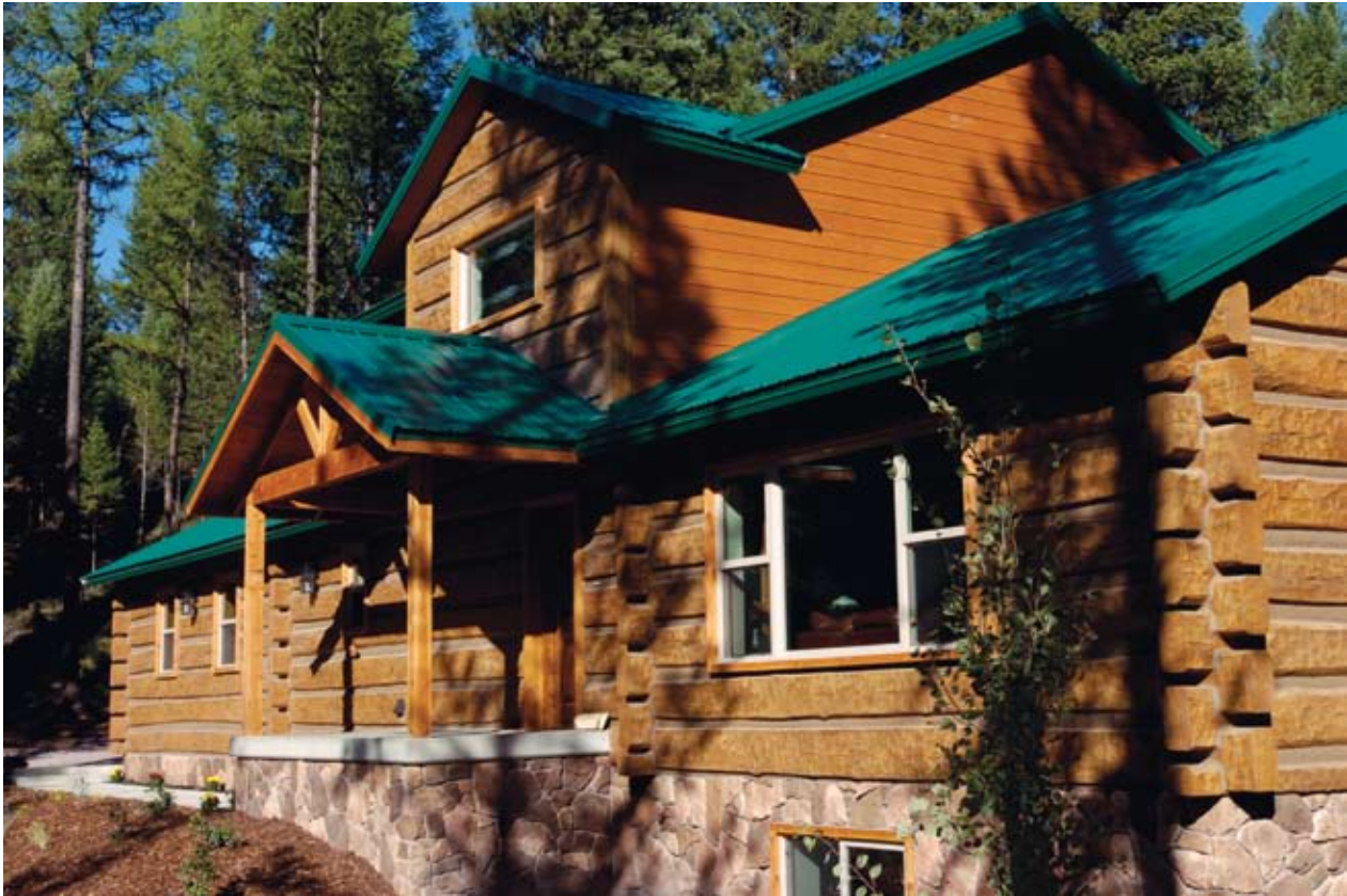
Precast Concrete Log Home, Missoula, Mont.; Architect: Beaudette Consulting Engineers with Cultured Log Systems; Photo: Cultured Log Systems.
