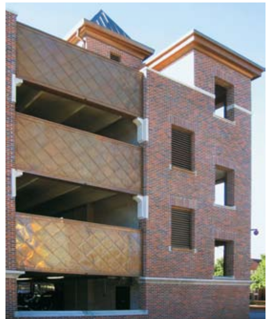
University of Denver College of Law Parking Structure, Denver, Colo.; Architect: University of Denver School of Architecture.
