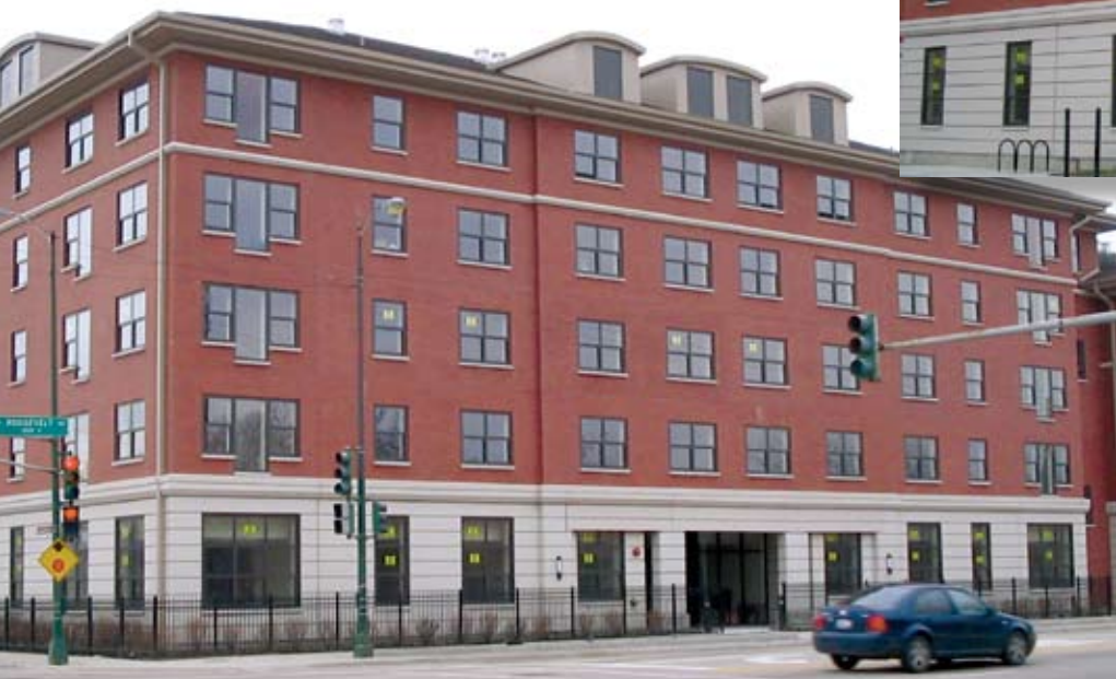
Roosevelt Place, Chicago, Ill.; Architect: Piekarz Associates PC; Photos: Prestress Engineering Corp.
