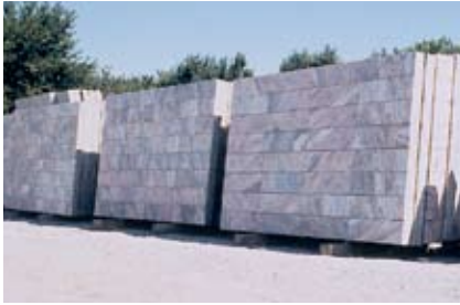
Architectural precast panels for the new wing of the Joslyn Art Museum, Omaha, Neb., are clad in Georgia marble to match the original stone building constructed in 1931. Labor and material cost were reduced using this system compared to traditional stone cladding systems. Architect: Henningson, Durham & Richardson Inc.
