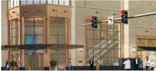
Stone veneer at the base of the 1700 Seventh Ave. building in Seattle adds an appropriate contextual detail.
