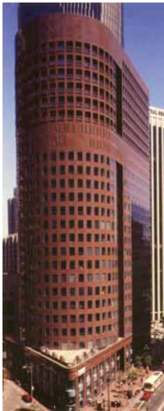
388 Market Street building in San Francisco, Calif. is clad with 3 cm granite anchored to precast concrete. (Architect Skidmore Owings & Merrill)
