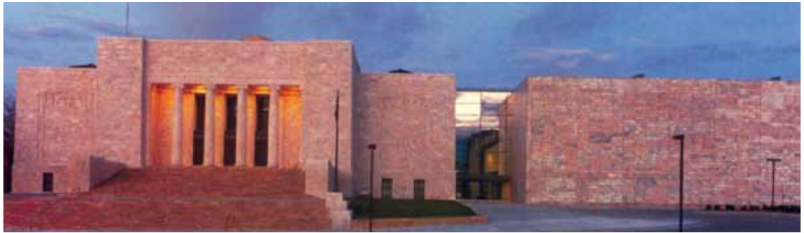
The new wing for the Joslyn Art Museum, Omaha, Neb. has 3 cm marble with 6 3 / 4 inch concrete backup. (Architects Sir Norman Foster and Partners; Architect of Record: Henningson, Durham & Richardson, Inc.)
