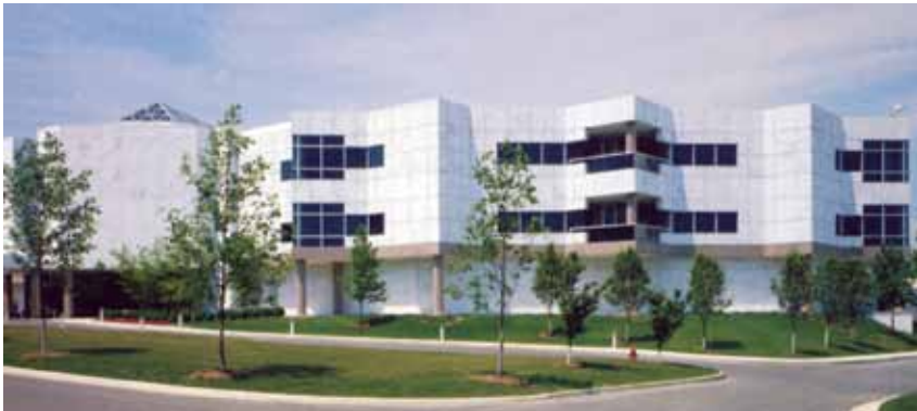
Hospital Corporation of America's Data Center, Nashville, Tenn. has 1 inch thick marble on a 5 inch precast concrete backup. (Architect Gresham, Smith and Partners )
