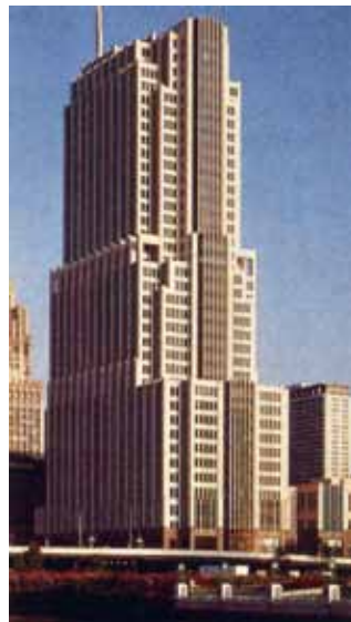
NBC Tower at Cityfront Center, Chicago, Ill. has 2 or 2 3 / 4 inch thick limestone on 5 inch thick precast concrete backing. (Architect Skidmore, Owings & Merrill)
