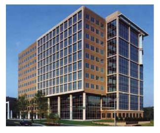
**Figure 18** Solid precast vertical pieces are used on the Glenridge Highlands One project in Atlanta to define the corners and the transitions from curtain wall to precast at the corners. Originally planned as returns and channel spandrel covers, they were cast solid at the precaster's suggestion for economy and detailing simplification.
