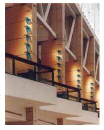
Figure 13 The returns on these column enclosures at the McCormick Place Expansion project in Chicago aren't intended to imply a material thickness of panels or blocks but to provide a planar wrap of the surfaces forming the corner. The joint is located at the pier's center to provide a linear continuation of the element above the pier.
