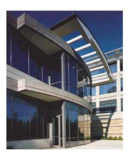
**Figure 14** In the smaller-scale detail provided at the ADP Building, Atlanta, a two-stage casting and dry-joint corner provide an abrupt but continuous return of the plane of the curvilinear sweep to the building face.
