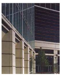
**Figure 10** On Chicago's McCormick Place Expansion project.,one-piece channel-shaped covers with relatively shallow returns were used to imply a thickness somewhat more than the actual panel thickness. In this case, well- executed "sharp" corners in the casting add to the solid appearance.
