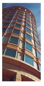
**Figure 12** This flat wall plane on the 55 Farmington building in Hartford, Conn., changes direction without corner articulation by using a shallow angle return for single casting and placing the joints at the back angles where they are de-emphasized. The shallow corner angle allows a solid cast edge.
