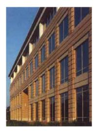
**Figure 9** The heavily rusticated panels used on 1335 Windward Concourse in Atlanta are thickened flat panels with exaggerated 3-inch quirks at the corners to create a return back into the interior of the building, giving it a perceived dimension.
