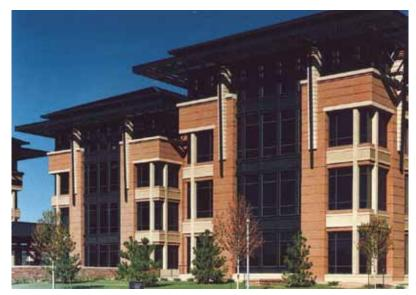
**Figure 11** Two-stage cast covers with deep returns were used for the solid-block treatments of piers at the Merrill Lynch Campus in Denver. The two-stage precasting allows a unique cast-in surface texture to be carried around the corners of the blocks to a much deeper dimension. Minimal corner dry joints without quirks complete the appearance of a solid unit.
