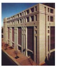
**Figure 16** The depth and shadowing of the façade on the Carrillon Building's parking structure in Charlotte, N.C., is continued in the detailing of the pier corners by using deep quirk miters to accent the corners with the shadow created by the larger quirk.
