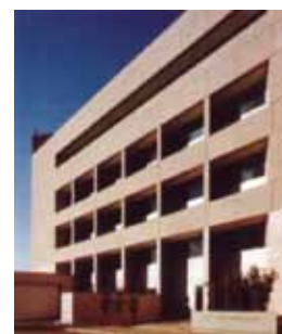
Figure 10 Deep recessed windows. (Courtesy © Glen Allison)
