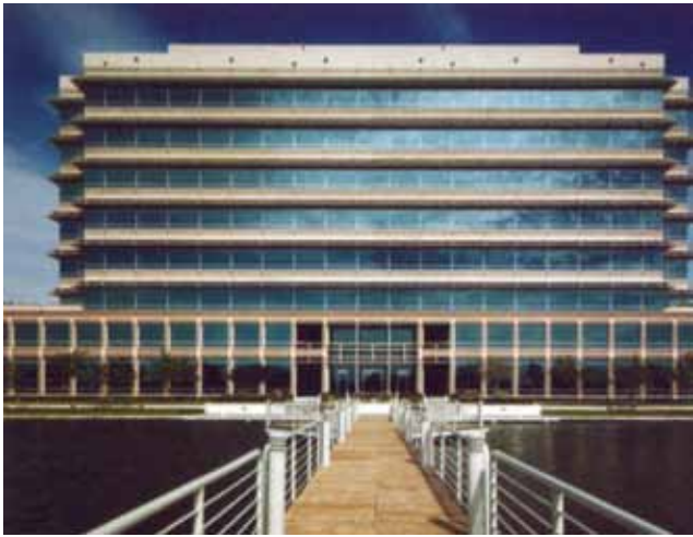
Figure 2 Horizontal sunscreen. (Courtesy © Brian Gassel/TVS & Assoc.)
