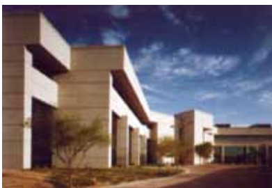
Figure 9 Cantilevered floor used to shade windows.
